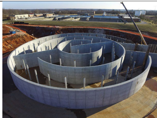
Dividing walls and columns
