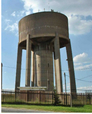
Circular, concrete, elevate storage
