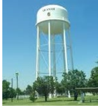
Circular, steel, elevated storage
