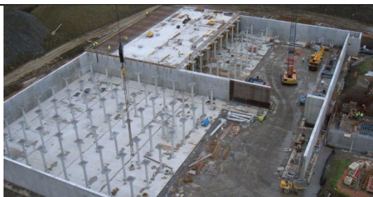
Internal support columns, concrete reservoir
