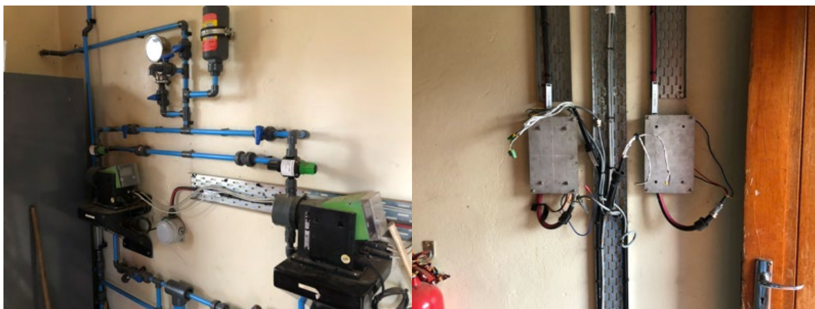
Figure 12: Ammonia dosing system
