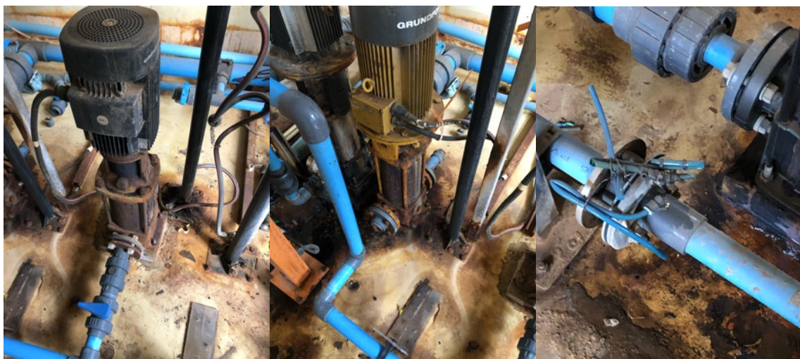
Figure 10: Poor condition of carriage water pumps
