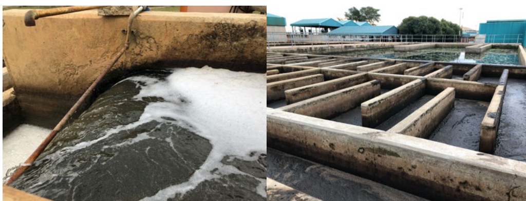
Figure 6: Module 4 flocculation and clarification
