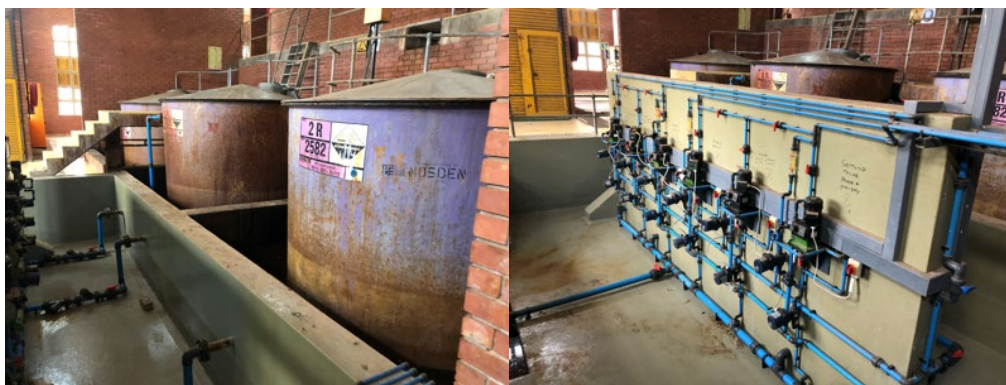
Figure 4: Polymer Day Tanks and Dosing Pumps
