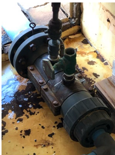
Figure 11: Leaking component (after chlorine injection)
