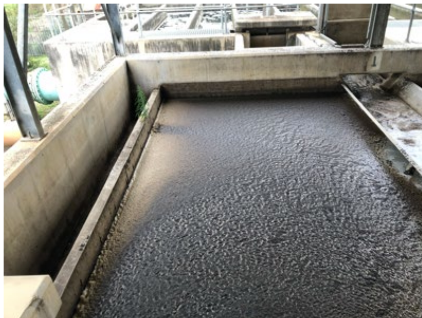
Figure 7: DAF unit for Module 5
