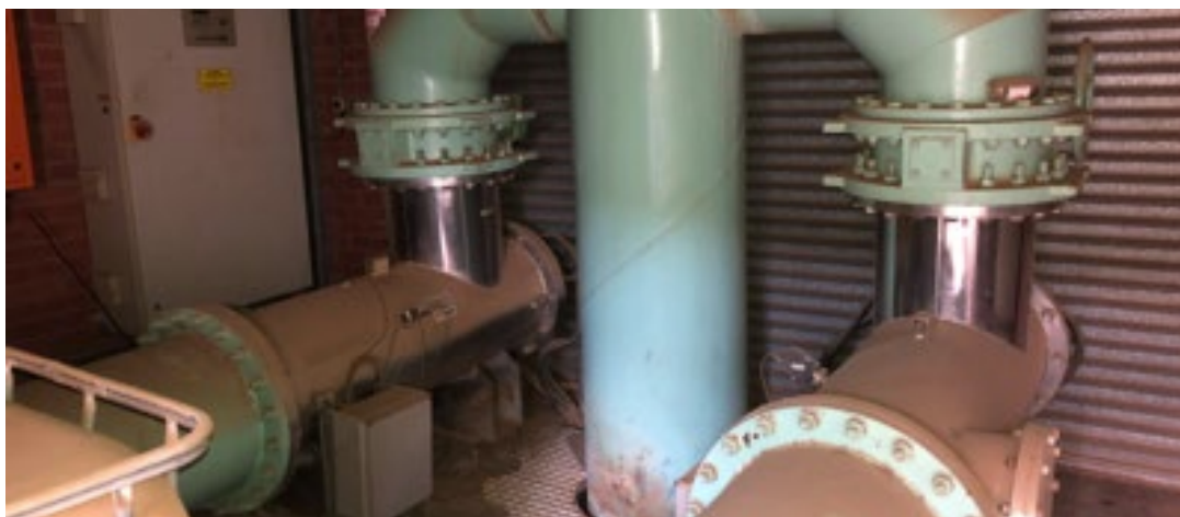
Figure 13: Ultraviolet System
