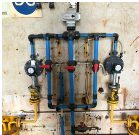
Figure 9: Change-over system but no second chlorine bank
