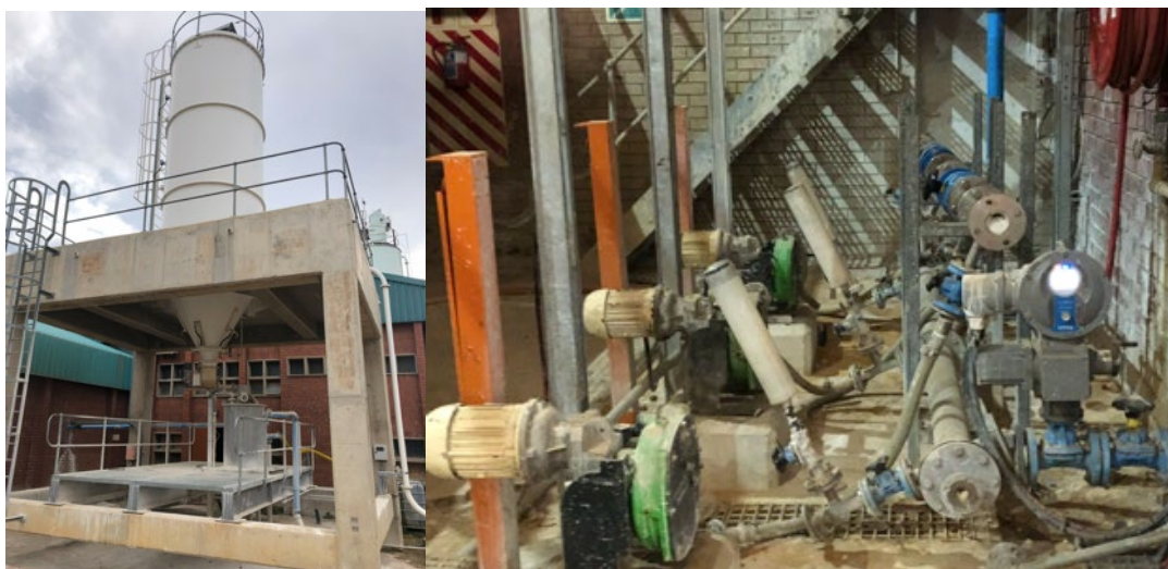
Figure 5: Lime dosing system (not operational)
