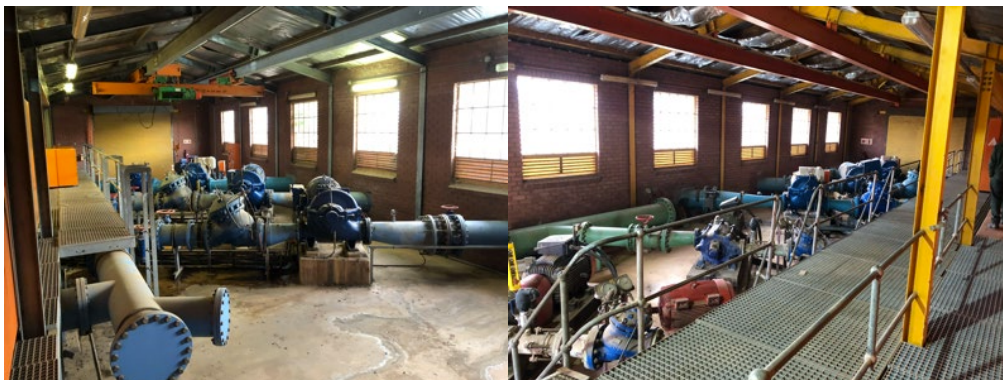
Figure 15: High Lift Pumps
