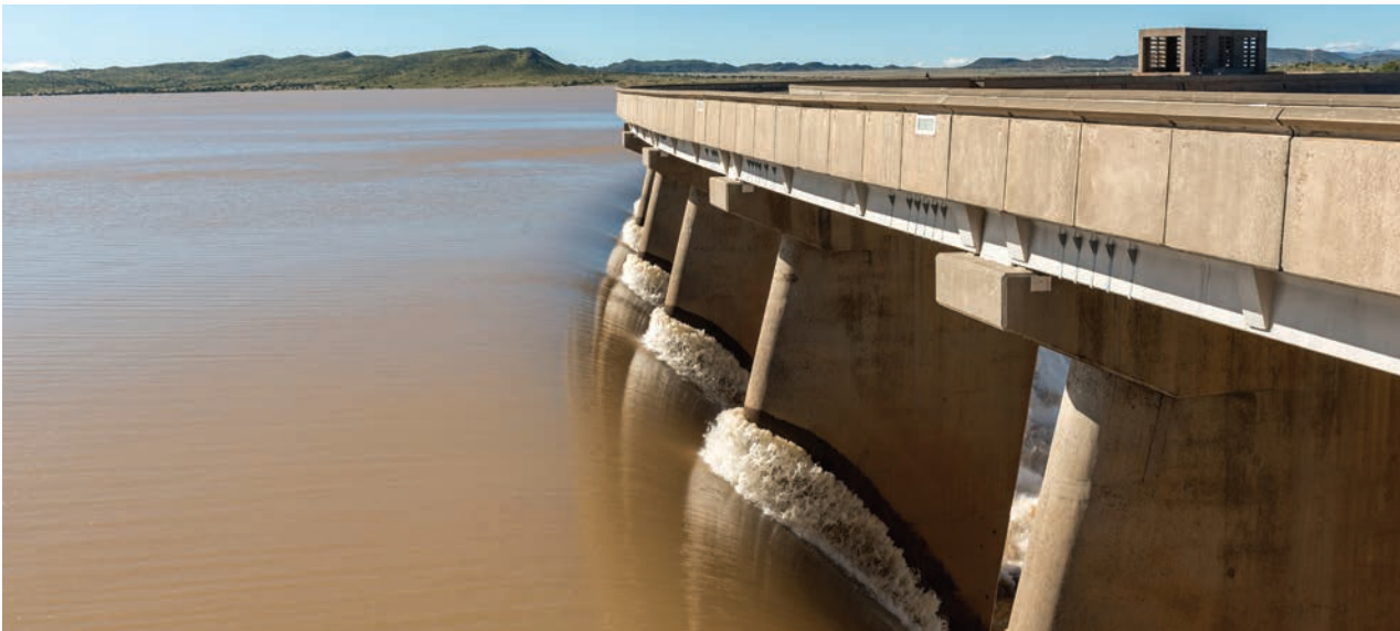
The Gariep Dam, in the Free State, is the largest dam in South Africa. Completed in 1972 the dam stores water from the Orange River. The dam wall is 88 metres high and contains about 1.73 million cubic metres of concrete. The dam has a capacity of 5 343 million cubic metres.
