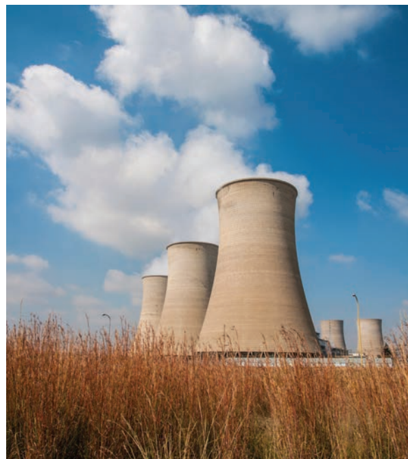
Power generation accounts for 2% of South Africa's freshwater use. The largest use of water in the energy sector is for cooling turbine exhaust steam.
