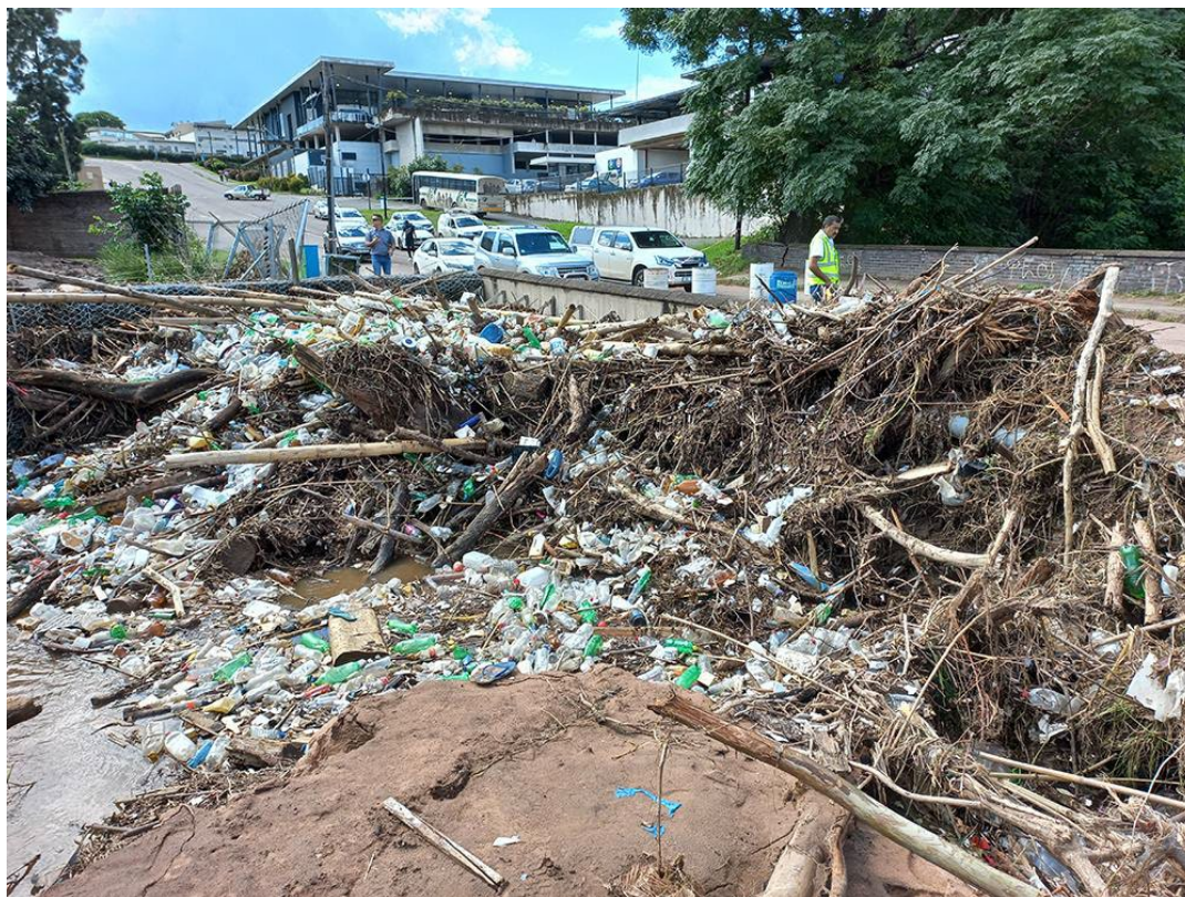
One of the many blockages caused by IAPs and solid waste in the 2022 eThekweni floods, resulting in damage to infrastructure and to services at and adjacent to the road crossing (Source: Geoff Tooley, eThekweni Municipality)
