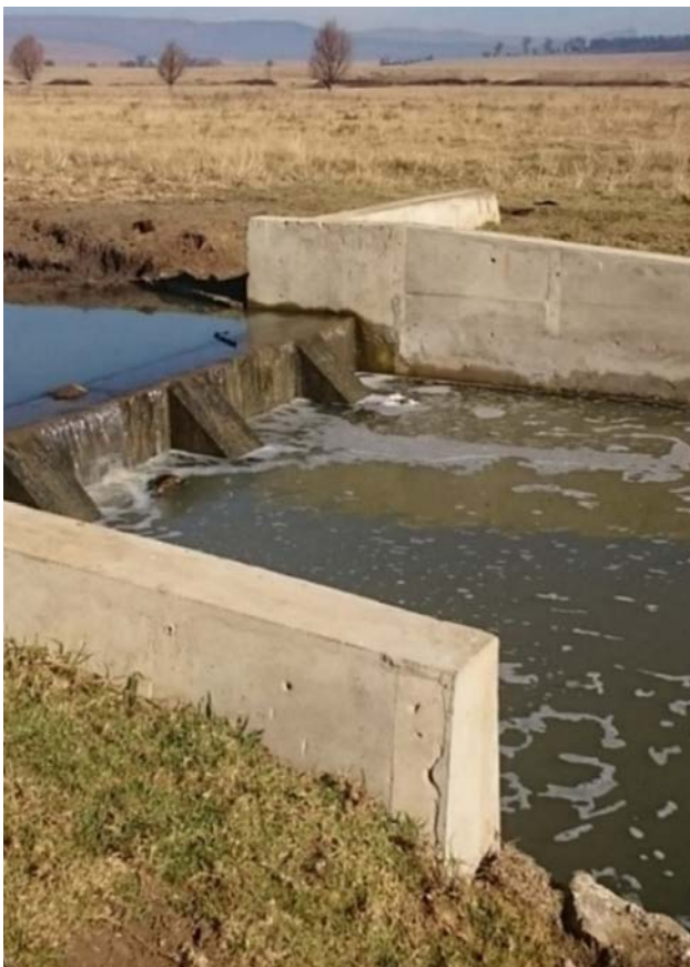
Concrete buttress weir built during phase 1 of Working for Wetlands construction cycle.
