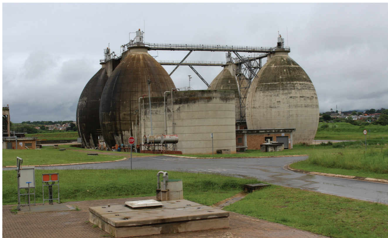
The anaerobic digesters, the Darvill works' most visually striking feature. Inside the heated eggs, bacteria break down organic waste in the absence of oxygen.
