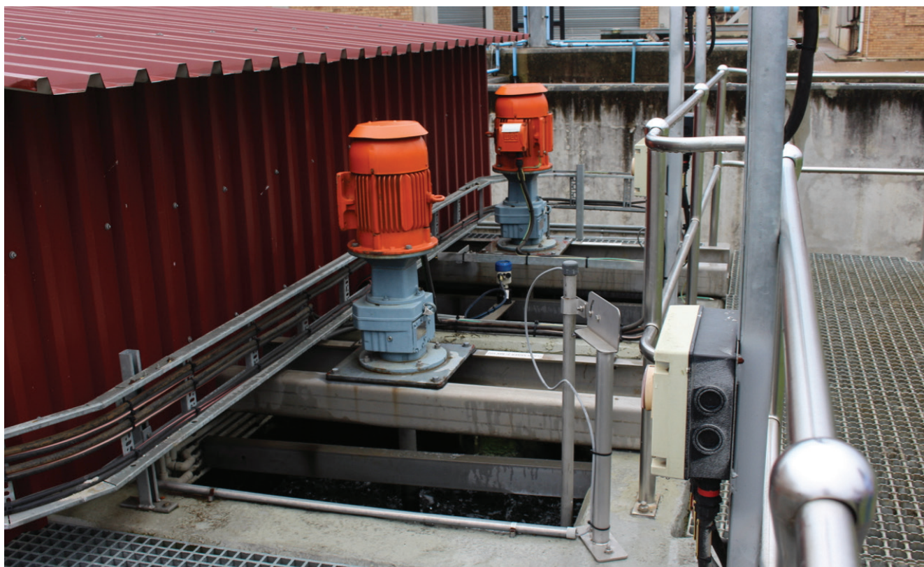
Flash mixing in the high-pressure wash plant disperses coagulants – aluminium sulphate and a polymeric coagulant – in the feed water. This helps suspended particles to clump together.
