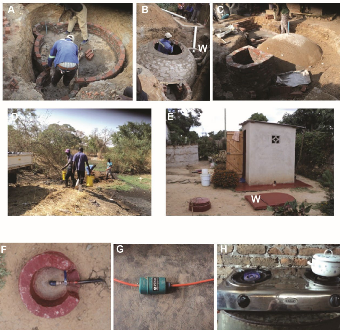
FIGURE 4-3: A SEQUENCE OF BIOGAS DIGESTER DEVELOPMENT STARTING FROM (A) LAYING FOUNDATION, (B) AN ALMOST COMPLETE DOME-SHAPED BIO-DIGESTER. THE THREE MEN ON THE MID TOP PHOTO ARE STANDING ON THE SITE OF THE TOILET. THE PIPE FROM THE RECTANGULAR TOILET BOX CONNECTS TO THE BIO-DIGESTER, (C) A COMPLETED DOME-SHAPED BIO-DIGESTER WITH THE GAS DELIVERY PIPE AT THE CENTRE. (D) CATTLE RUMEN CONTENTS BEING LOADED ONTO THE LORRY AS A START-UP MATERIAL. THE RUMEN IS CO-DIGESTED WITH FAECAL MATERIAL FROM THE TOILET, (F). THE DELIVERY PIPE WAS CONNECTED TO A VALVE, WHICH IN TURN WAS CONNECTED TO THE GAS DELIVERY PIPE WHICH PASSED THROUGH A CONDENSER AND A (G) DE-SULPHURISER. (H) THE GAS IS CONNECTED TO A TWO-PLATE LPG GAS STOVE. NOTICE THE BLUE FLAME OF THE GAS ON THE LEFT PLATE.
