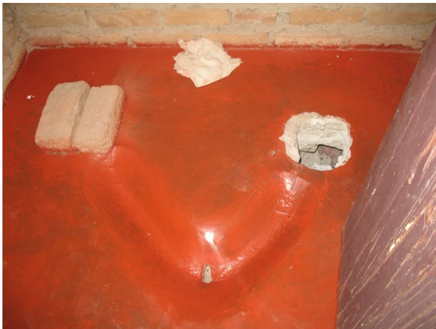
The two-hole urine diverting Skyloo interior
