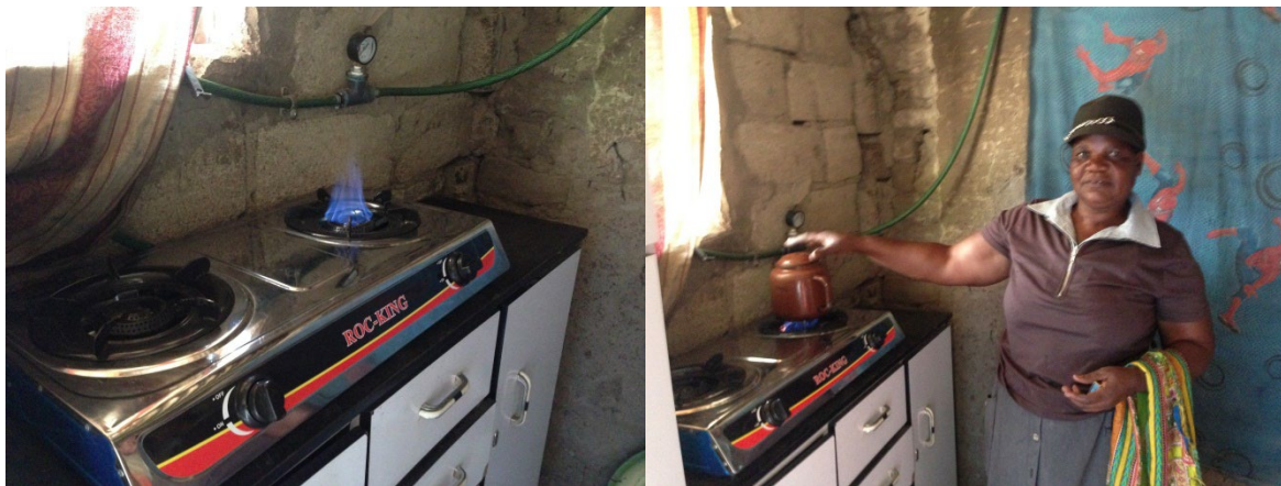
FIGURE 4-4: BIOGAS GENERATED FROM THE DIGESTER AT HOPLEY (LEFT) BEING USED FOR COOKING (RIGHT)
