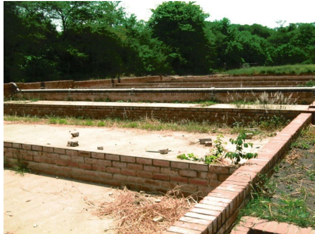
FIGURE 1-4: DRYING BEDS FOR SEWAGE SLUDGE (NOT IN USE)
