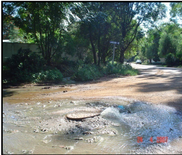
FIGURE 1-11: OVERFLOWING MANHOLE IN HARARE
