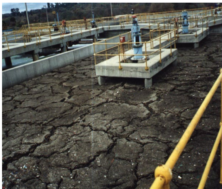
FIGURE 1-3: NON FUNCTIONAL BNR TREATMENT WORKS
