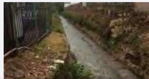
Canalised rivers have less capacity to deal with pollution as they lack plants that could take up or trap pollutants.
