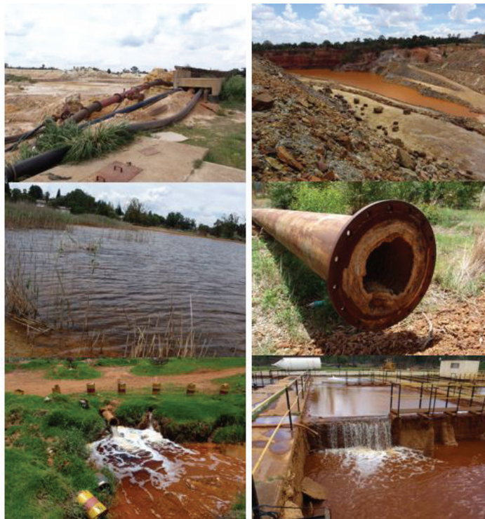
Figure 4-2: Acid mine drainage in the Tweelopiespruit, which shares a source area with the Wonderfonteinspruit. The headwaters area is dominated by mine dumps which pollute both streams.
