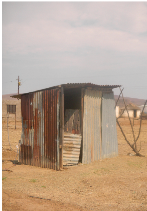
Typical village toilet (non-ventilated pit latrine)
