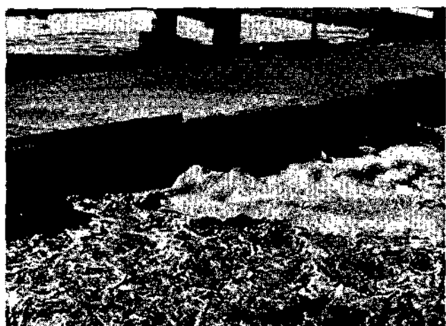
Figure 6c Lower side of picture showing scum being formed in aerobic zone and drifting through the barrier into the anoxic zone
