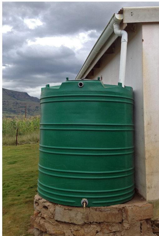
During rooftop water harvesting rainwater is simply collected from rooftops and stored in tanks.
