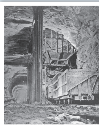
Left: The Orange Fish Tunnel during excavations.
