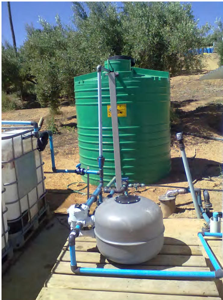
The olive wastewater storage and pretreatment unit.
