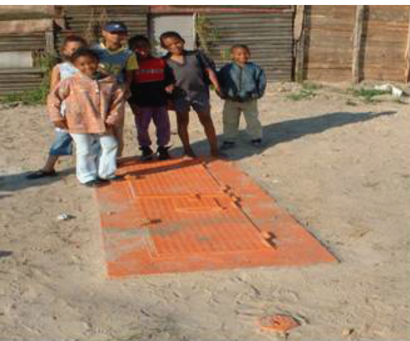
Figure A10. Orange colour coded treated effluent meter chamber
