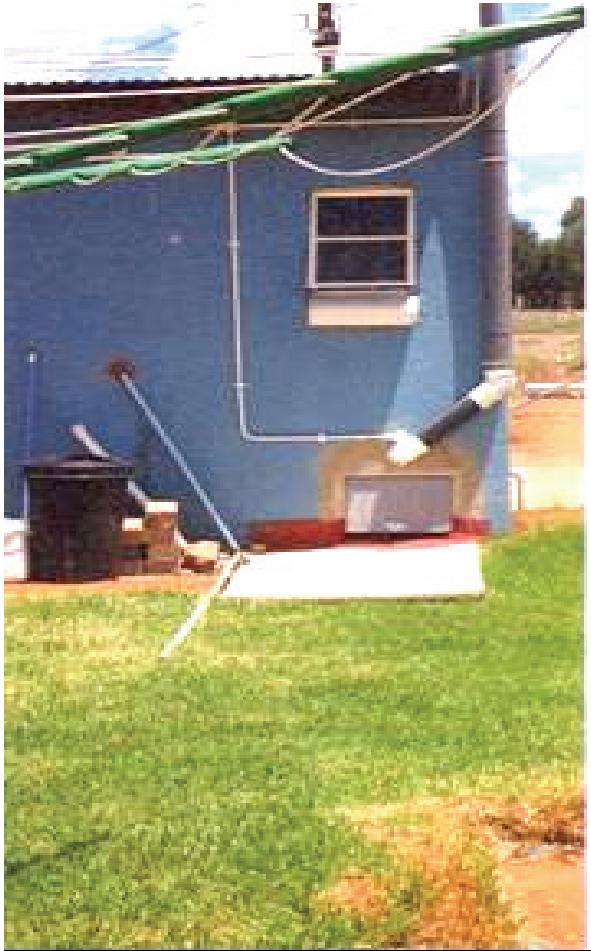
Figure 16. Above surface irrigation using washing machine grey water
