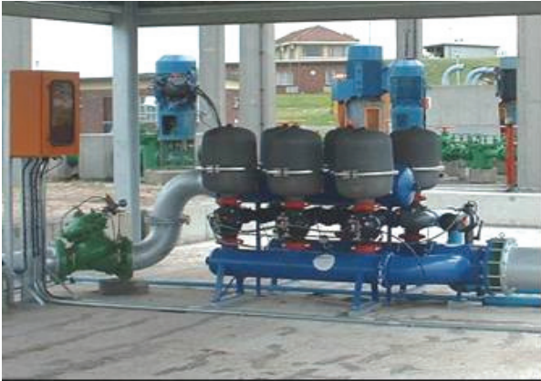
Figure A6. A modular filtration unit
