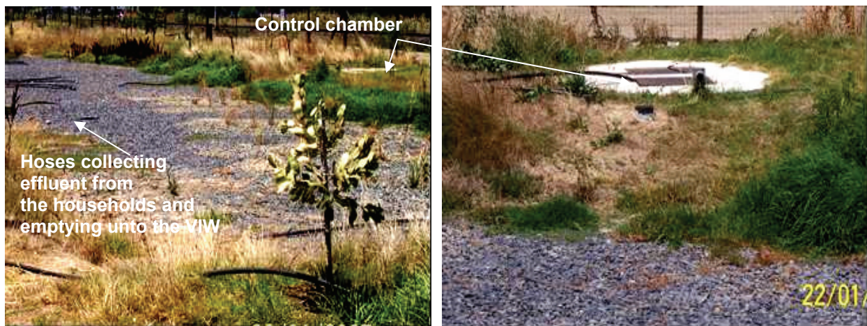
Figure 26. The Vertically Integrated Wetland and control chamber
