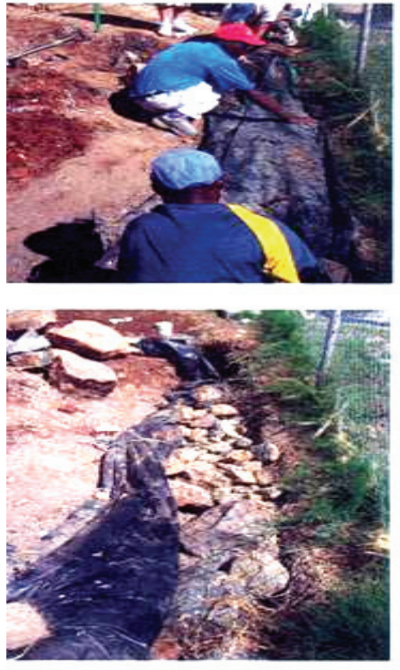
Figure 17. Below surface irrigation using kitchen grey water
