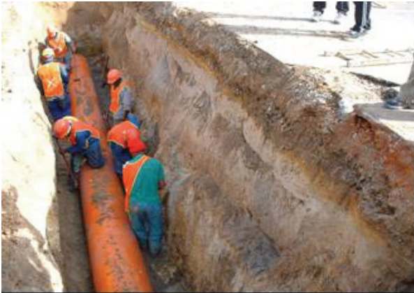
Figure A8. Orange colour coded 600 mm GRP treated effluent supply mains through Koeberg road
