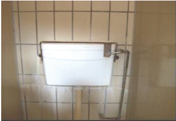
Figure 32. A communal toilet cistern supplied with treated effluent*
