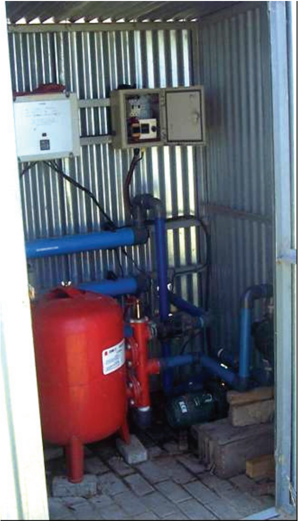
Figure 21. The ultraviolet unit
