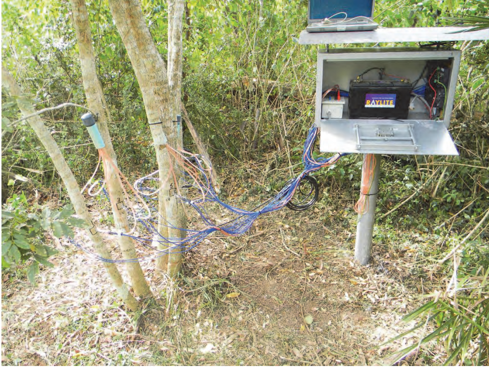
Figure 13. View of instrumentation that was installed, and the stems that were monitored, at the Umzimbeet site (Photo: M. Gush).
