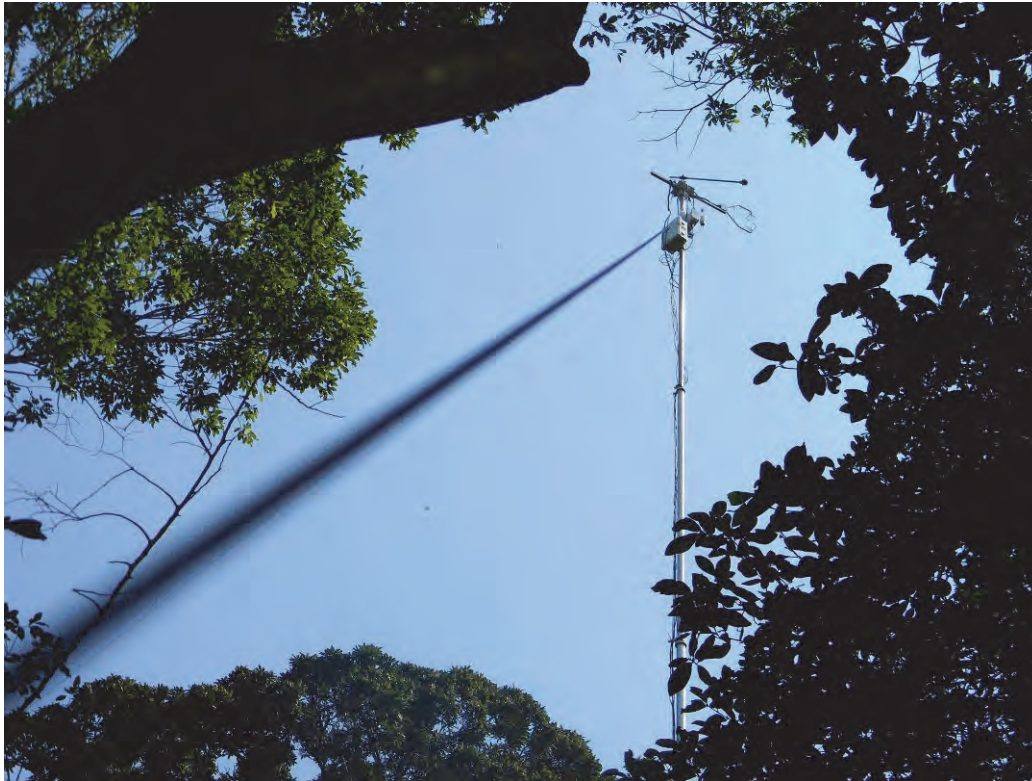
Figure 15. Fully installed telescopic mast projecting above forest canopy, with supporting guy ropes and mounted eddy covariance instrumentation (Photo: M. Gush).
