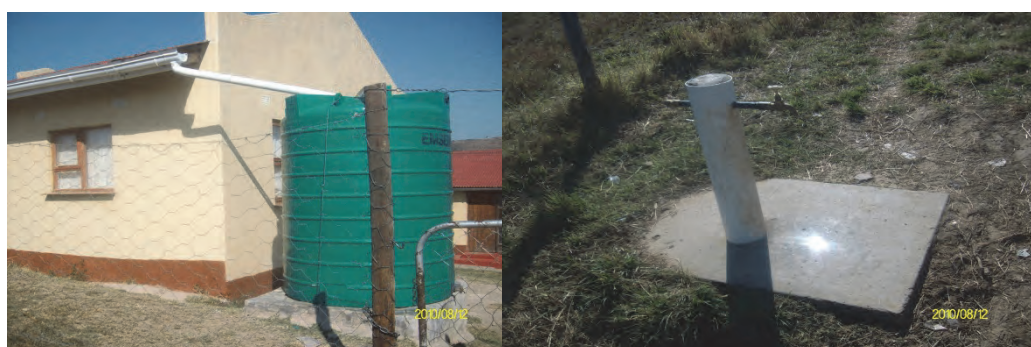
Figure 4.6 Water harvesting off roofs and a communal tap at Willowvale, Eastern Cape.
