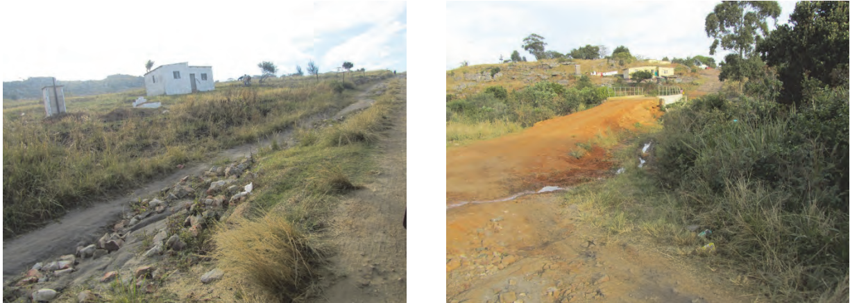
Figure 7.5 The poor condition of roads can be problematic and hinder marketing of produce at Marina, Eastern Cape.
