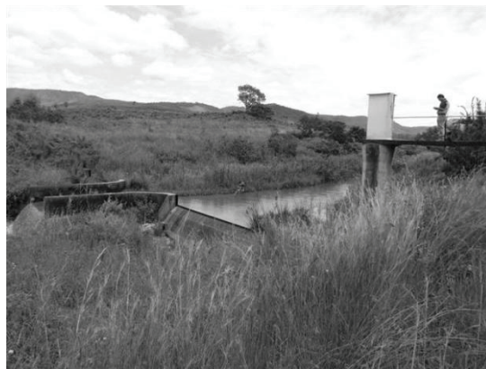
Figure 7.19 Flow gauging weir X2H024 (DWA, 2012)
