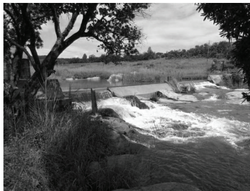
Figure 7.23 Flow gauging weir X2H008 (DWA, 2012)
