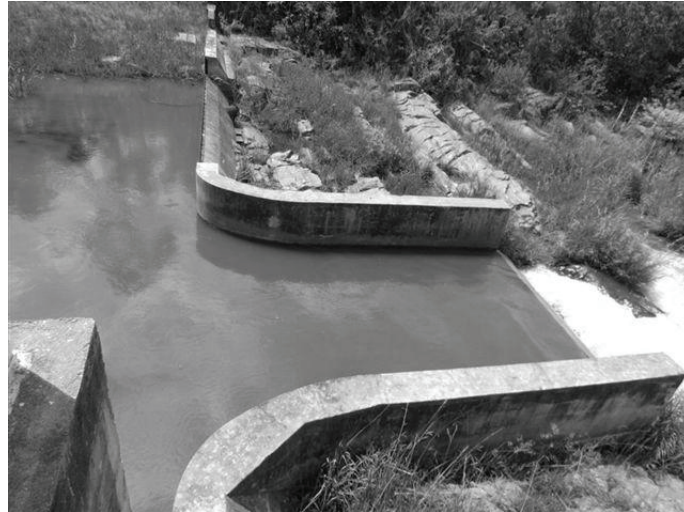
Figure 7.11 Flow gauging weir X2H010 (DWA, 2012b)
