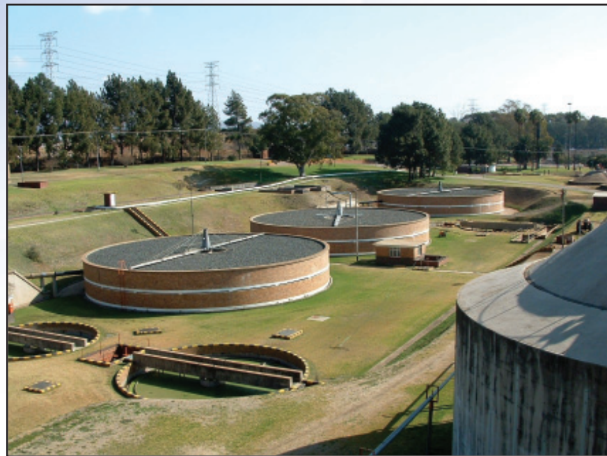
Aerial view of the previously decommissioned trickling filters at Daspoort Sewage Works
