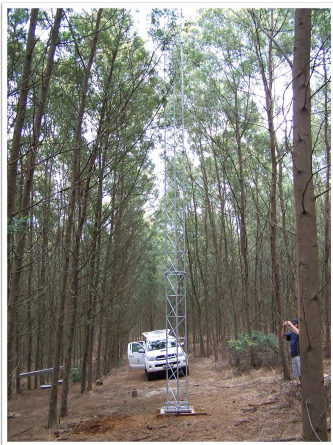
Figure 3.7: Base of the 24 m lattice mast in the centre of the Wattle tree stand. A hinged base-plate was concreted into the ground for stability.
