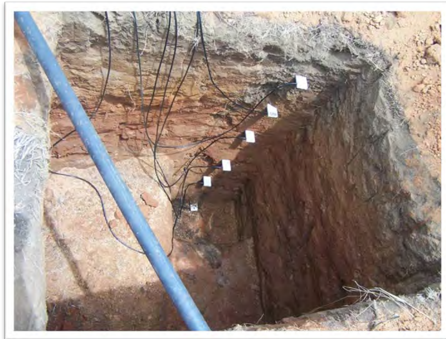
Figure 3.21: Pit excavated to a depth a 2.5 m near the lattice mast at Two Streams for the installation of CS616 probes at 0.4 m intervals.
