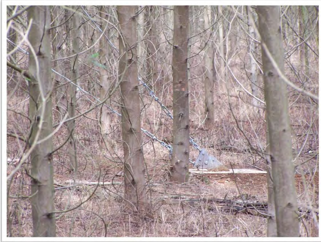
Figure 3.9: The steel guys were secured onto custom brackets that were concreted into the ground.
