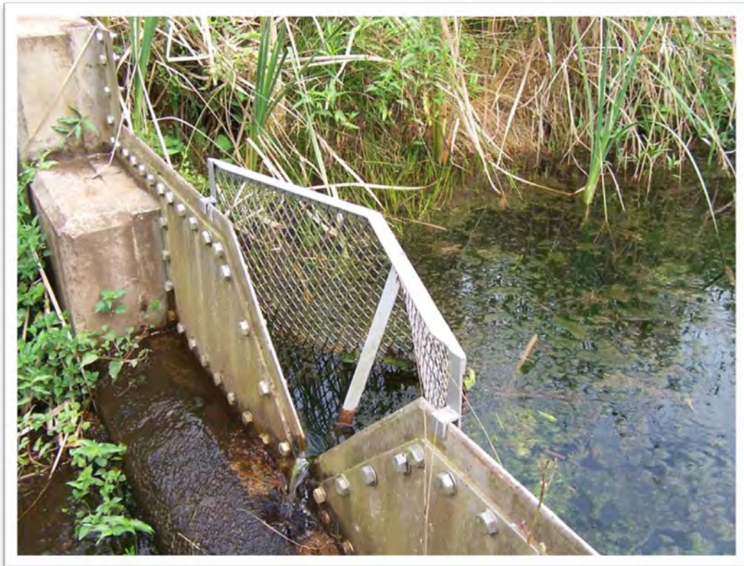
Figure 3.17: The new sieve in the main weir at Two Streams in 2011 prevents blocking of the V-notch which affects water level results.
