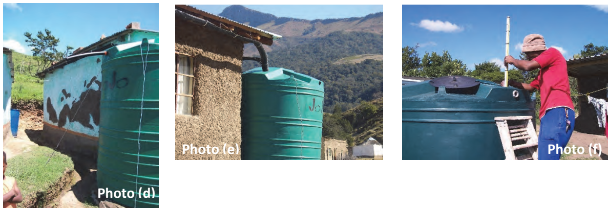
Above and below: Photos of Lutengele roofwater harvesting and agric-training. Photos (d) and (e) collection from traditional houses using flexible guttering, (f) Leak-proof testing, (g) diversion-swailes in gardens, (h) training in mulching and contouring, (i) trench beds and diverse crops.
