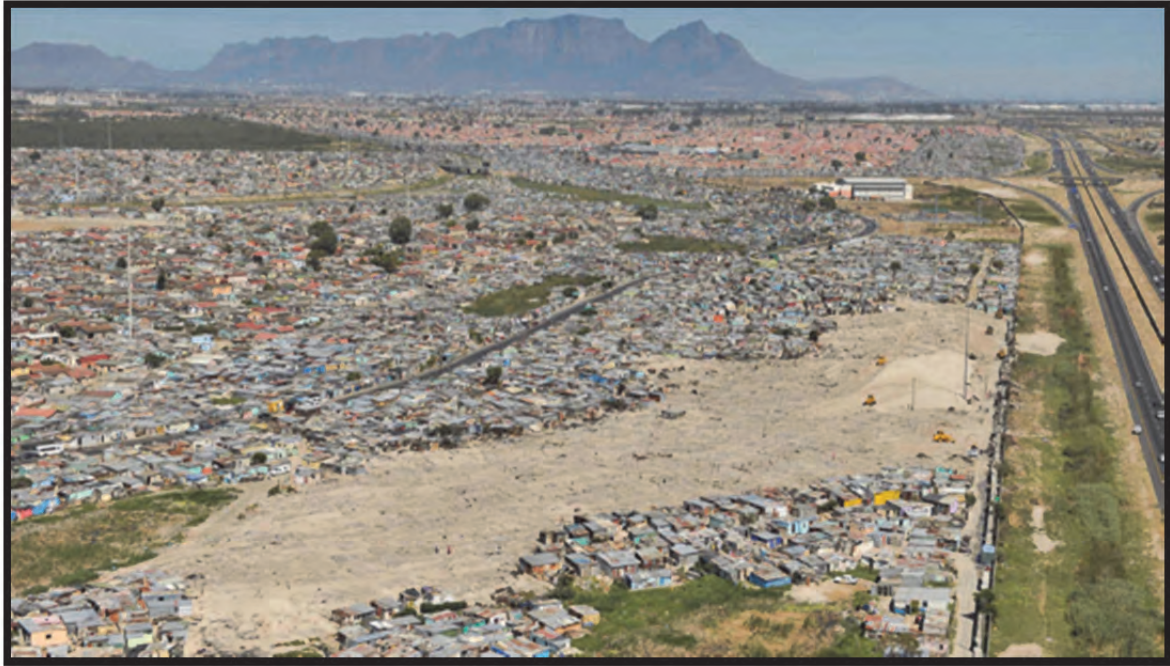
Figure 3-6: BM Section after a devastating fire (Photo by CoCT, 5 January 2013).
