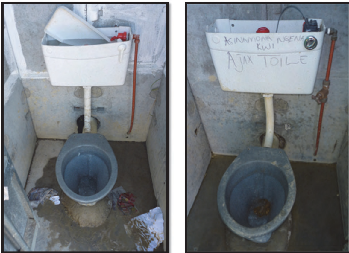
Figure 3-11: A toilet in "good working condition" (left) versus a toilet in "bad working condition" (right). Both toilets notably do not have toilet seats or operational flush levers, but the former was considered "good" because it discharges wastewater into the sewer as intended, whilst the latter does not.
