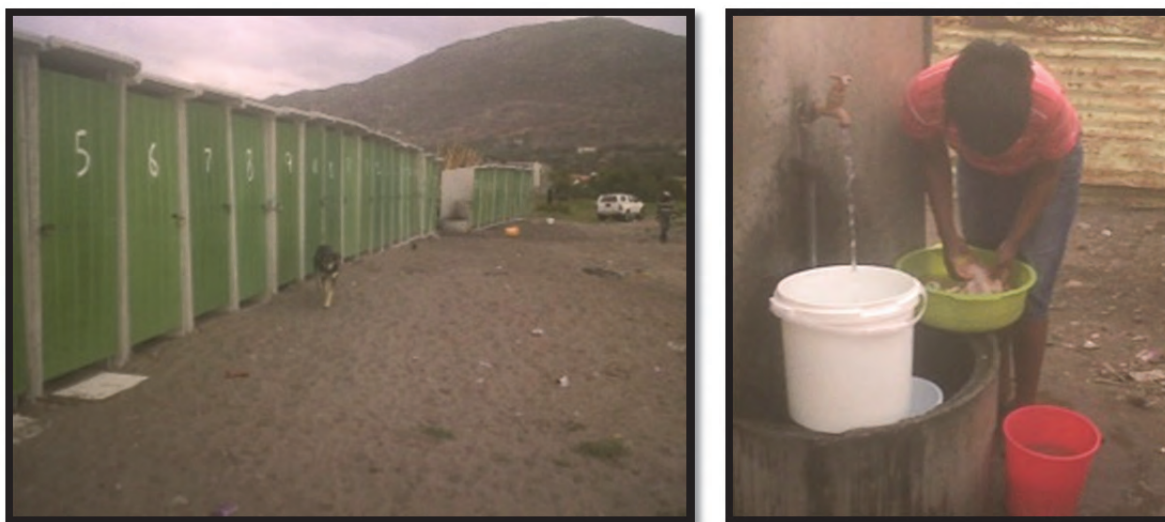
Figure 3-18: E-Section toilets (left) and a woman washing clothes at one of two standpipes in E-section (right) (Schroeder, May and June 2013). Of the 36 toilets there, only 1 was unlocked.
