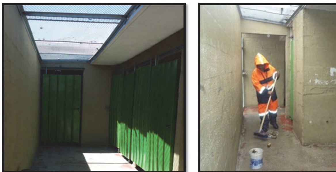
Figure 4-9: BM ablation block's metal grid ceilings allow for natural light (left), and rain and wind (right) (Taing, February and July 2013). A janitor cleans the ablation block facility in full rain gear on the right.
