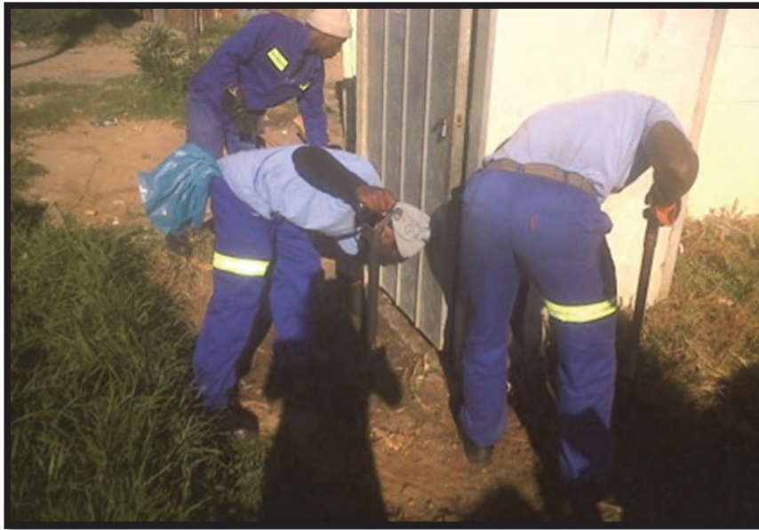
Figure 3-23: Janitors digging trenches and clearing overgrowth in the TRA (Schroeder, May 2013).
