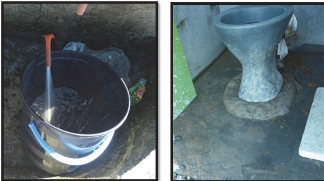
Figure 3-26: In general, the water and sanitation infrastructure along the N2 in BM Section needed to be replaced. On the left is a broken water pipe that a woman said she "unbent" whenever she needed water and to the right is a broken discharge pipe from which newspaper and faecal matter emanated (Taing, May and June 2013).
