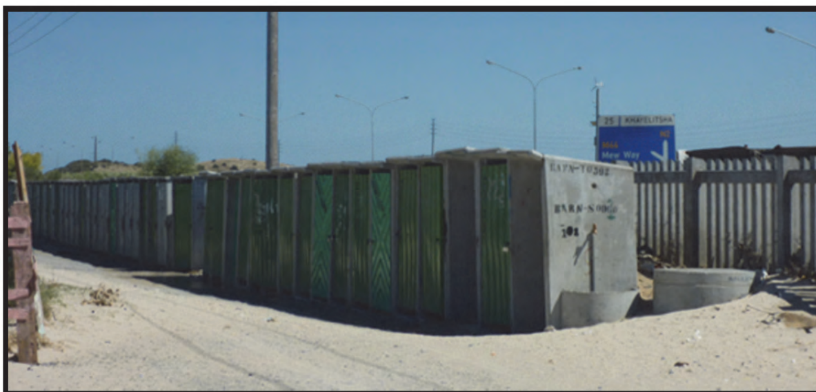
Figure 3-9: A cluster of toilets in BM Section alongside a dirt and gravel road that is covered with a layer of sand (Taing, February 2013).
