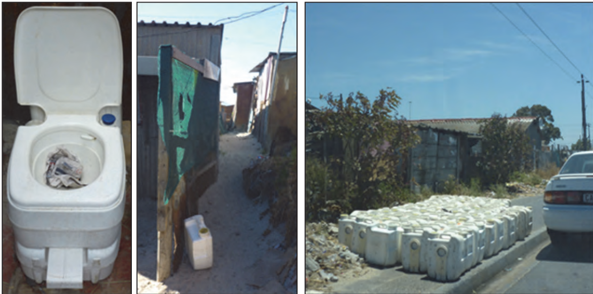
Figure H-2: A porta-potty in BM Section (left); a tank that is to be collected by the porta-potty service provider (centre); and 'cleaned' tanks left on Lansdowne Road by the service provider for users to pick-up (right) (Taing, January-March 2013).
