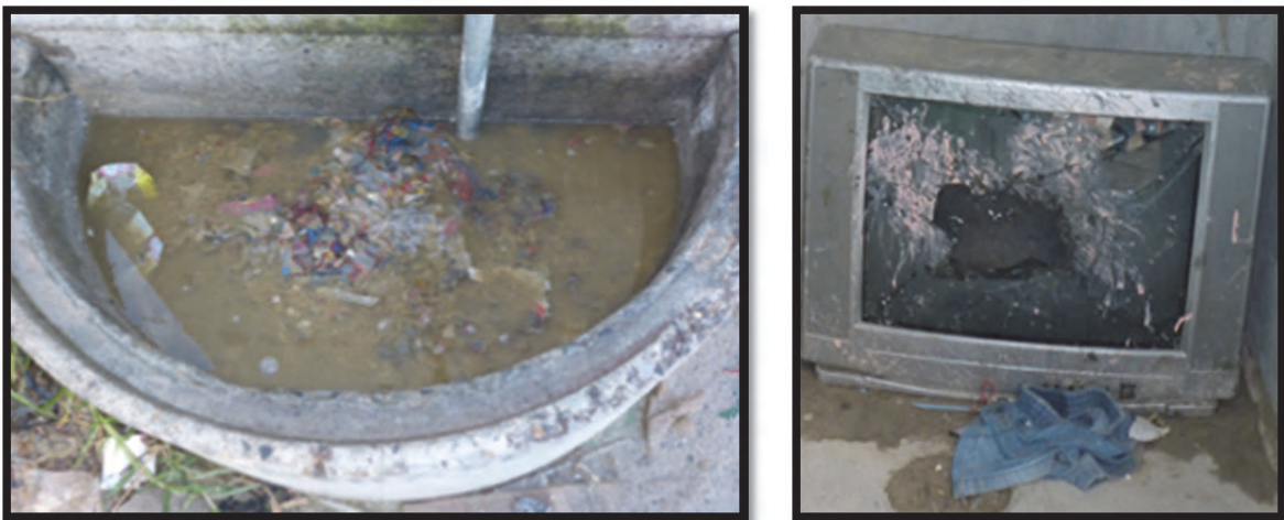
Figure 4-11: The lack of drainage for household wastewater in BM Section often meant that residents dumped their buckets of night soil and greywater into gullies of communal standpipes (left), which is also where some collected their household water. Residents also disposed of refuse in toilet cubicles (right) (Taing, January 2013).
