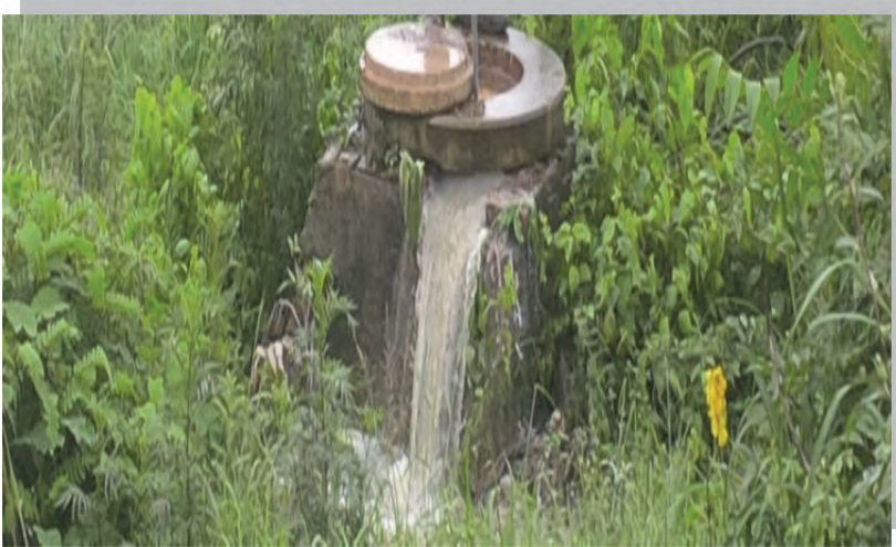
Figure 4.1. A blocked sewage main draining into Msunduzi River
