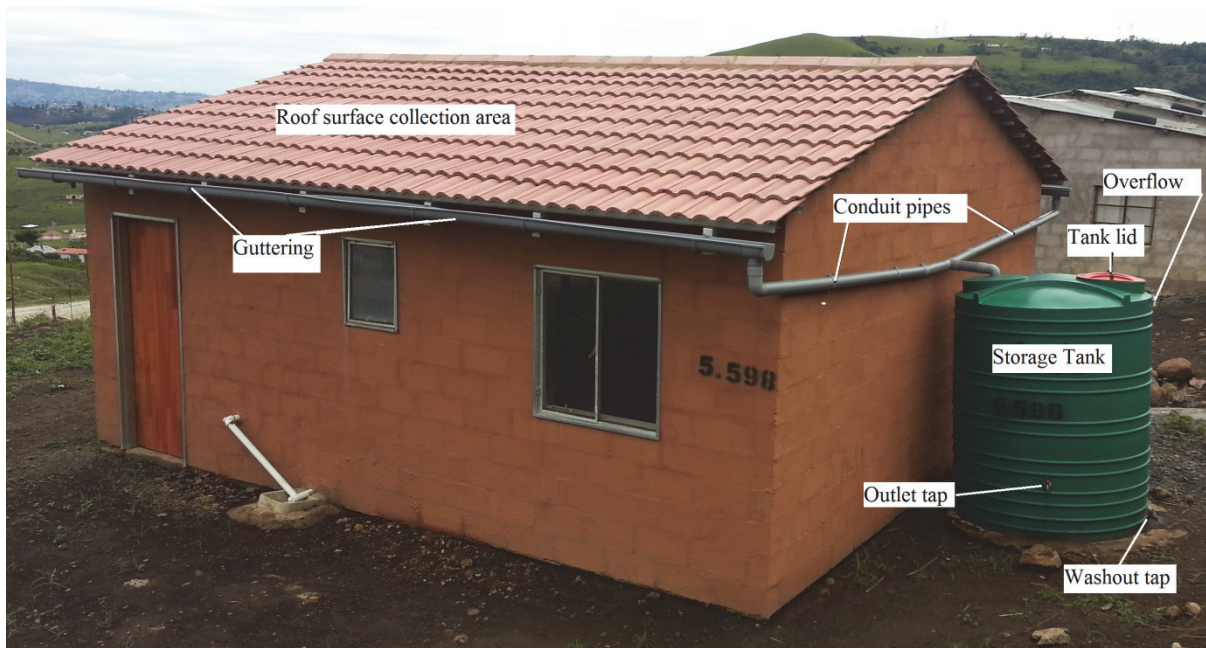
Figure 2.1 A typical rooftop rainwater harvesting system.
