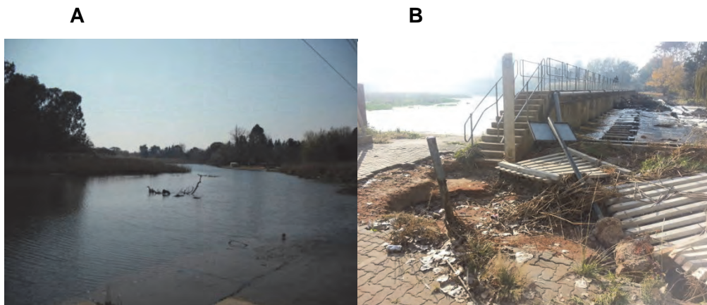
Figure 19: Site photographs of Klip River 4 showing (A) upstream and (B) downstream.
