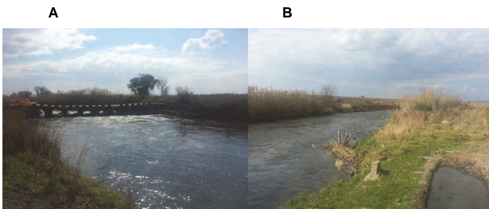
Figure 18: Site photographs of Klip River 3 showing (A) upstream and (B) downstream.
