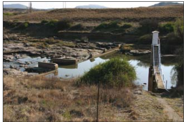
Figure 16 Example of a Hydro flume in combination with a sharp-crested weir in the Kraai River catchment (Eastern Cape)
