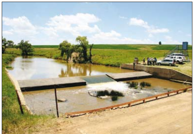
Figure 9 Example of a horizontal compound Crump weir without dividing walls in the Vaal River catchment (Mpumalanga)
