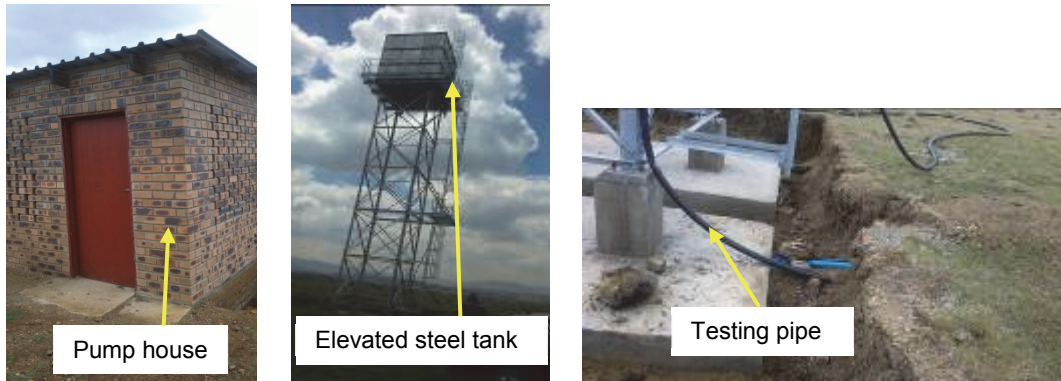
Figure 3.30: Charlestown community water system photos
