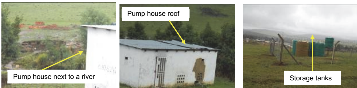
Figure 3.20: Msawawa community water system photos
