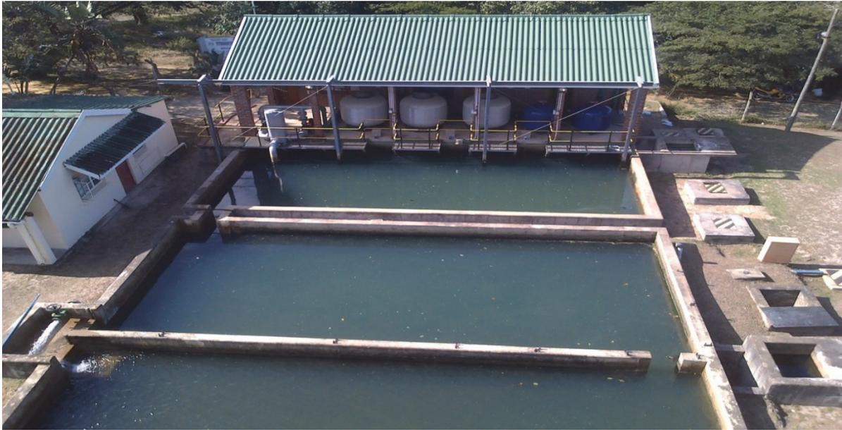
Figure 138. View of the three water sedimentation tanks at the Mbazwana WTW and the five sand filters used in the early treatment process.
