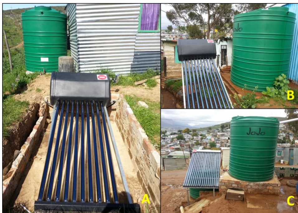
Figure 4.1. Two small-scale rainwater harvesting solar pasteurisation treatment systems were installed at Mr Victor Mthelo's home [Site 1 (A)] and Pastor Makhaya Qondani's church [Site 2 (B)], respectively. A large-scale rainwater harvesting solar pasteurisation treatment system was installed at the ERC [Site 3 (C)].
