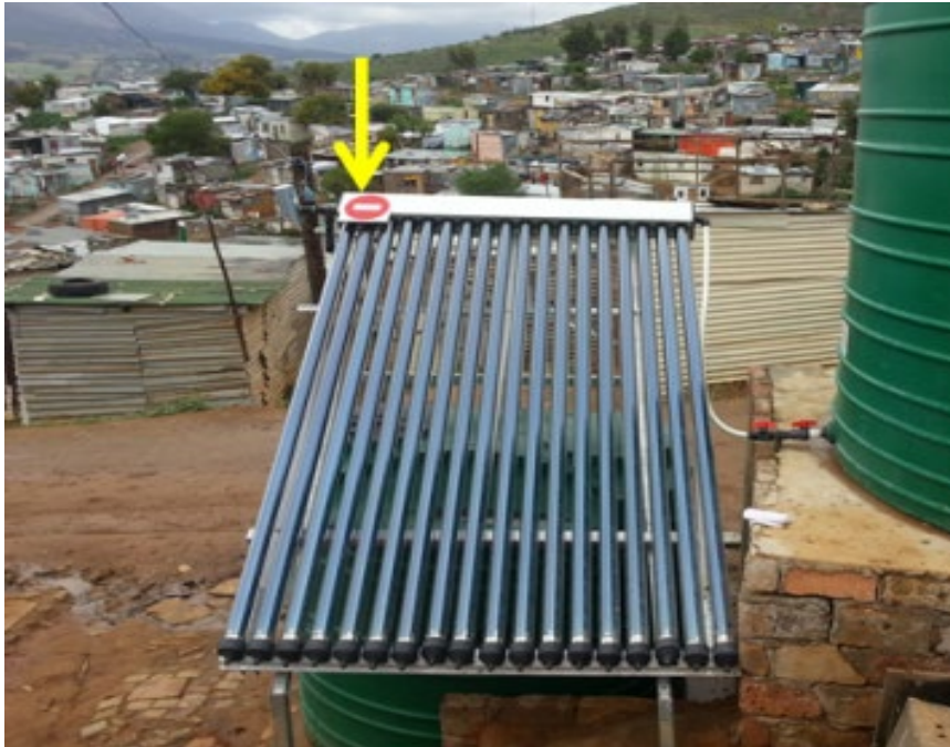
Figure 4.17. The solar pasteurisation system connected to the rainwater harvesting tank at the ERC (Site 3). The “NO ENTRY” sign is attached to the manifold as the solar pasteurisation system does not have a storage unit. The treated rainwater thus flows into a holding tank.
