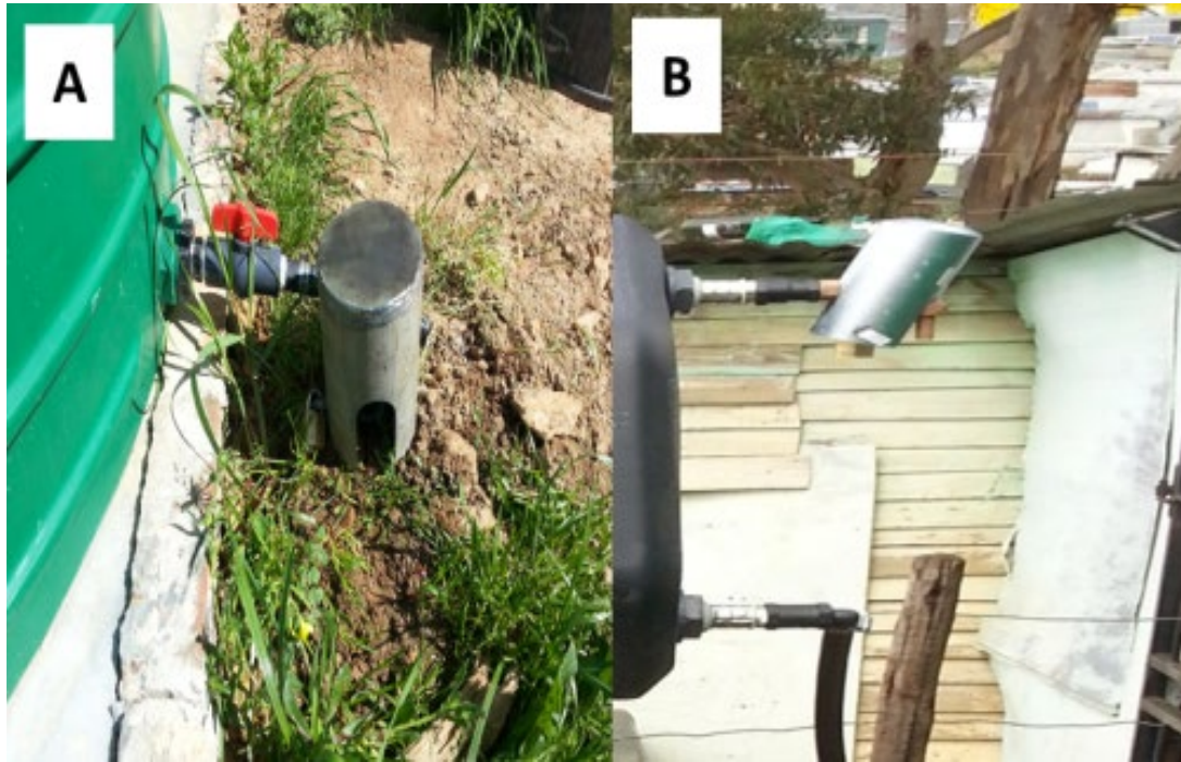
Figure 4.11. The taps connected to the rainwater harvesting tanks (A) and storage units of the solar pasteurisation systems (B) are locked. For this reason each household was provided with a set of keys for the respective latch locks.
