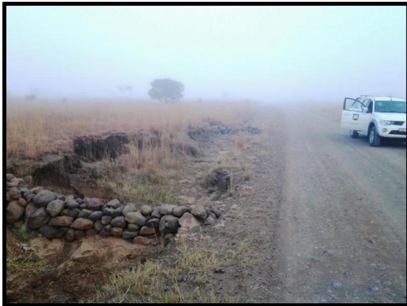
**Figure 2-28: Efforts to stop erosion along the road (Located at Photo 7 in Figure 2-3).**
