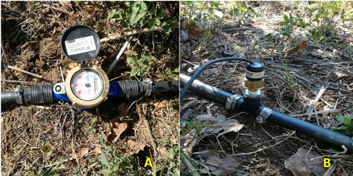
**Figure 3.11 Layout of irrigation monitoring and soil water sensors in the intermediate and mature orchards. A) water meter, B) pressure switch**
