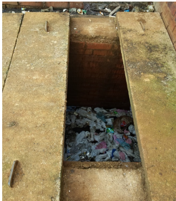
Figure 45: A pit cover panel was missing behind the girls' toilets, presenting a serious safety threat
