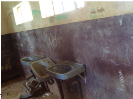
Basins in the girls' toilets before (left) and after (right) renovation. Basins were reattached and taps and water supply piping installed. However, with the position of the taps, and the holes on the top of the basins, water often dripped through the holes, creating large puddles on the floor and making access to the toilets difficult.
