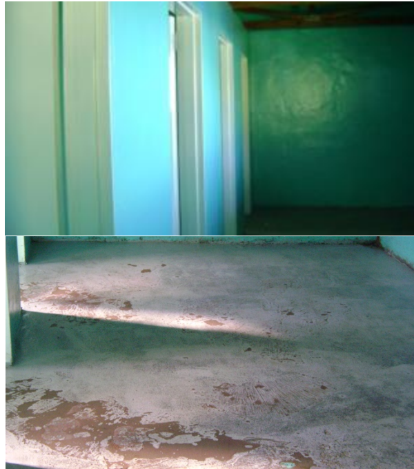
Figure 13: New paint for walls and floors at School B – The walls and floors were both painted. The paint used on the floor was meant to seal it and make it easier to clean, but the HSO reported that when he tried to clean the floors, the paint simply chipped away, leaving the floors constantly looking dirty.
