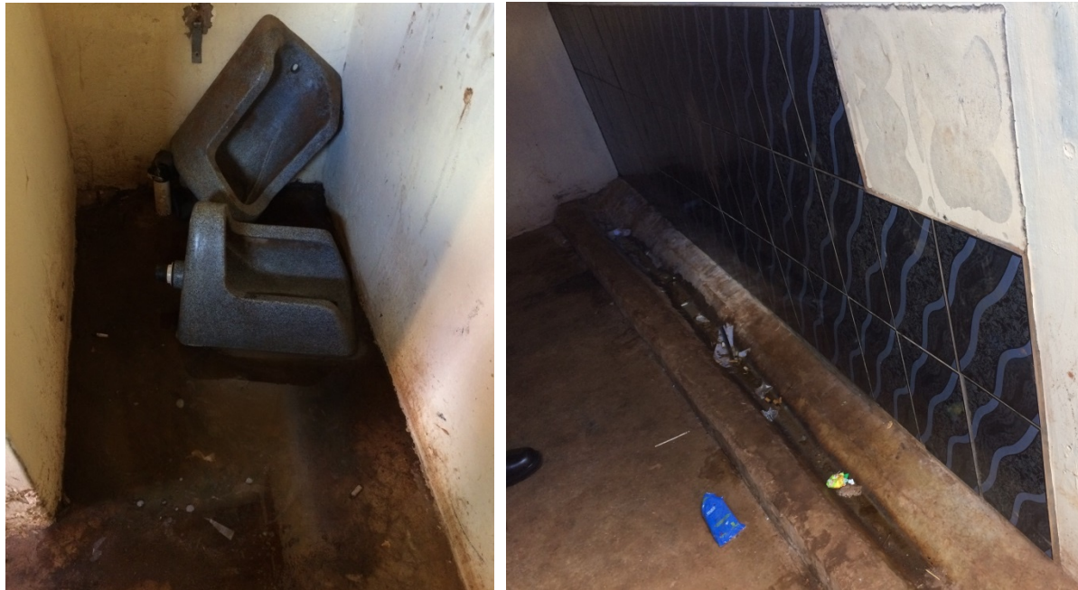
Figure 56: State of boys' urinals at School F before launch – wall-mounted urinals removed from the wall and a puddle of urine (left); and the trough urinal, with tiles installed by the contractor, but very shallow and without adequate slope to provide drainage of urine
