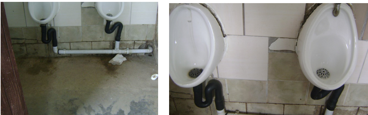
Figure 29: New wall-mounted urinals were installed and misused, leading to large amounts of urine on the floor most of the time; the mounting on the wall also appears to be inadequate (right), causing the HSO to fear that the urinals would fall off the wall.
