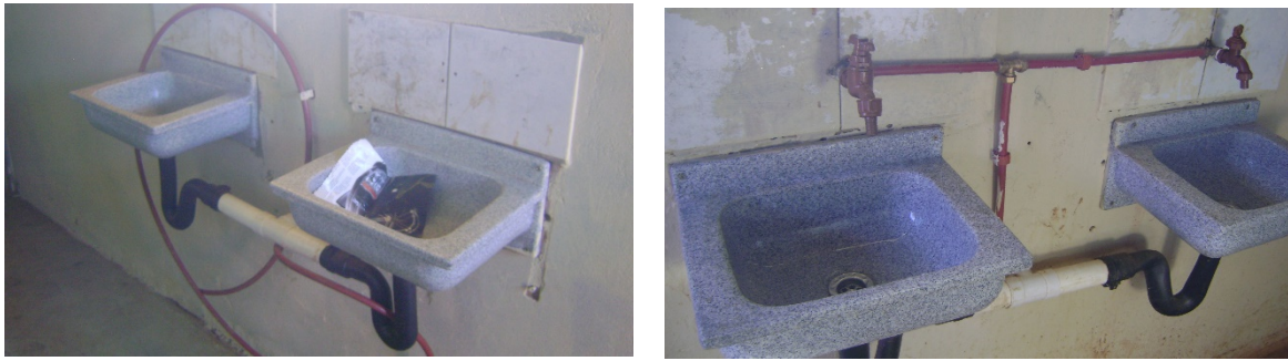
Figure 38: The contractor initially departed with the basins in an unfinished state (left), but came back after a substantial delay to complete installation of taps and water pipes.
