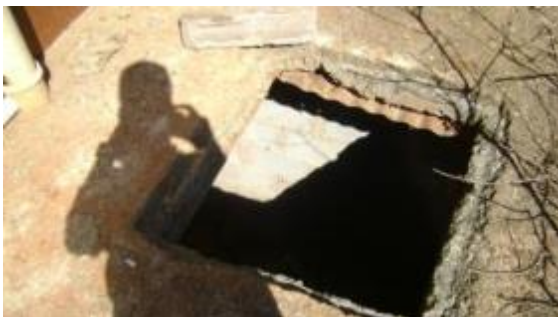
Pit covers (left) were not repaired or replaced, and old Phungalutho toilets (right) were not demolished.
