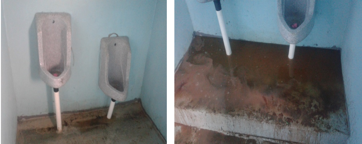
Figure 11: New urinals at School B – The contractor sealed the floor urinal trough and installed two wall-mounted plastic urinals in its place. The HSO expressed great dissatisfaction with this change, partly since the learners were not used to these types of urinals and also because it reduced the number of “urination spaces” from as many as could fit along that wall to only two. This led many learners to urinate on the floor, out of previous habit or necessity, and there was no longer any drainage for the urine.
