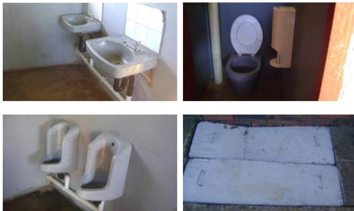
Figure 34: Department upgrades to School G sanitation – (upper left) Handwashing basins were connected and taps installed; (upper right) toilet seats were replaced; (bottom left) urinals in the boys’ toilets were installed correctly and connected; (bottom right) the contractor installed a new pit cover, but it was not properly reinforced and had begun breaking before the programme had launched
