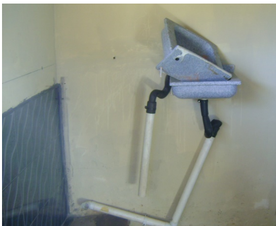
Figure 48: Basins not properly re-installed in the boys' toilets
