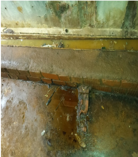
Figure 46: A urinal with inadequate drainage
