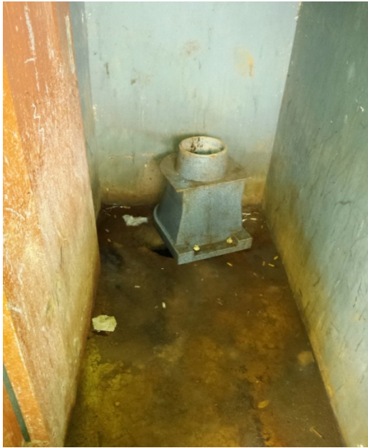
Figure 42: A pedestal removed from the slab above the pit
