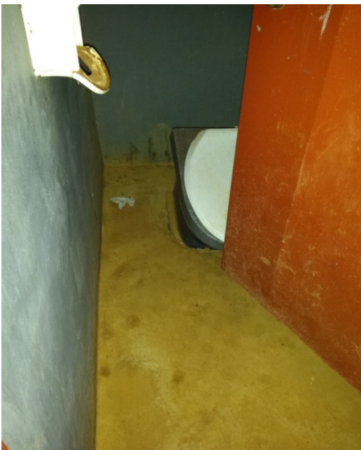
Figure 44: A portion of the slab in a girls' toilet stall was collapsing, presenting a serious safety threat
