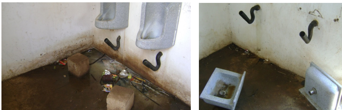
Figure 70: Urinals and basins at a KZN Primary School – photos taken just 3 years after the toilets were built
