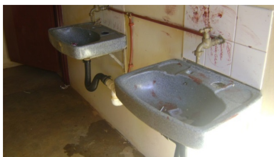
Figure 52: The taps were installed too close to the wall, such that water spills on the basin sill and does not fall into the basins
