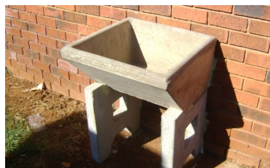
Figure 53: Outdoor basin installed with no water connection or tap
