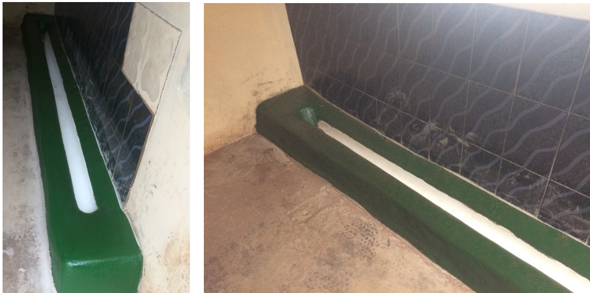
Figure 57: School F renovated urinal – improved using a gutter sloped to the drain and painted with water-resistant epoxy
