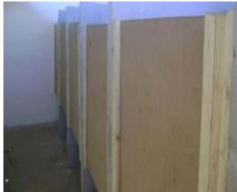
Figure 24: The doors installed in the girls' upper block were inadequate, since they did not reach the floor and were positioned high off the ground. They also were not equipped with locks, which further limited the degree to which they would afford girls the intended privacy.
