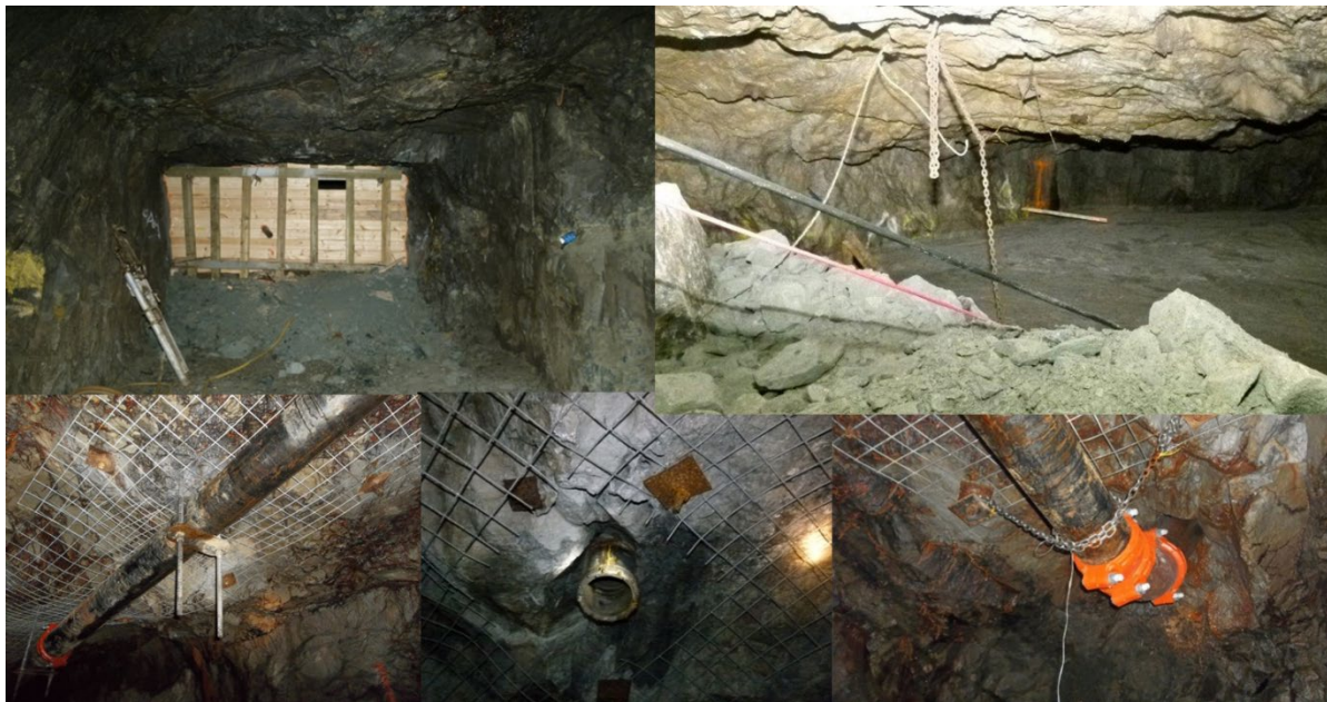
Figure 2: Cemented paste backfill operations at Giant Mine (Golder, 2018)
