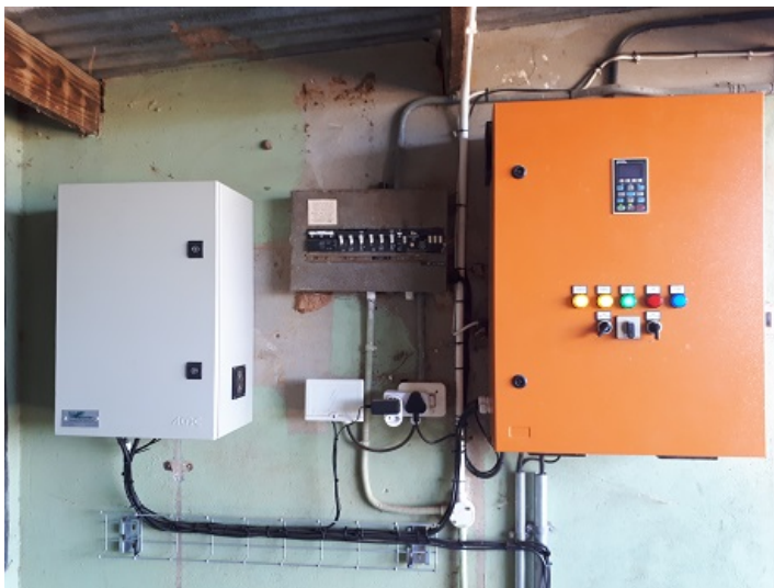
Figure 21: Many of the farmers have installed Variable Speed Drives (VSDs) to their pump stations. These automatically ensure that the right amount of pressure is used per block. This saves a significant amount of energy, as well as water.
