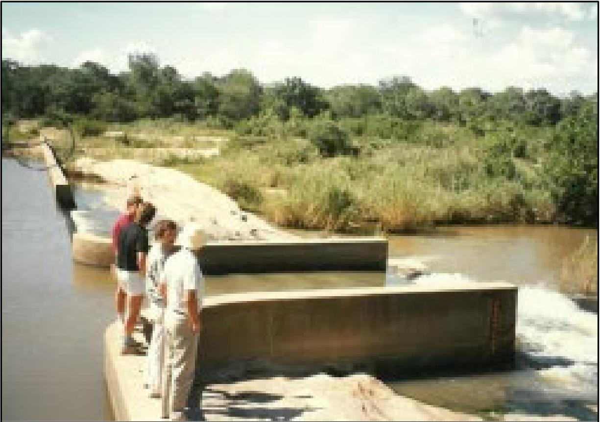
**Figure 7.17:** Compound gauging-weir X3H008
