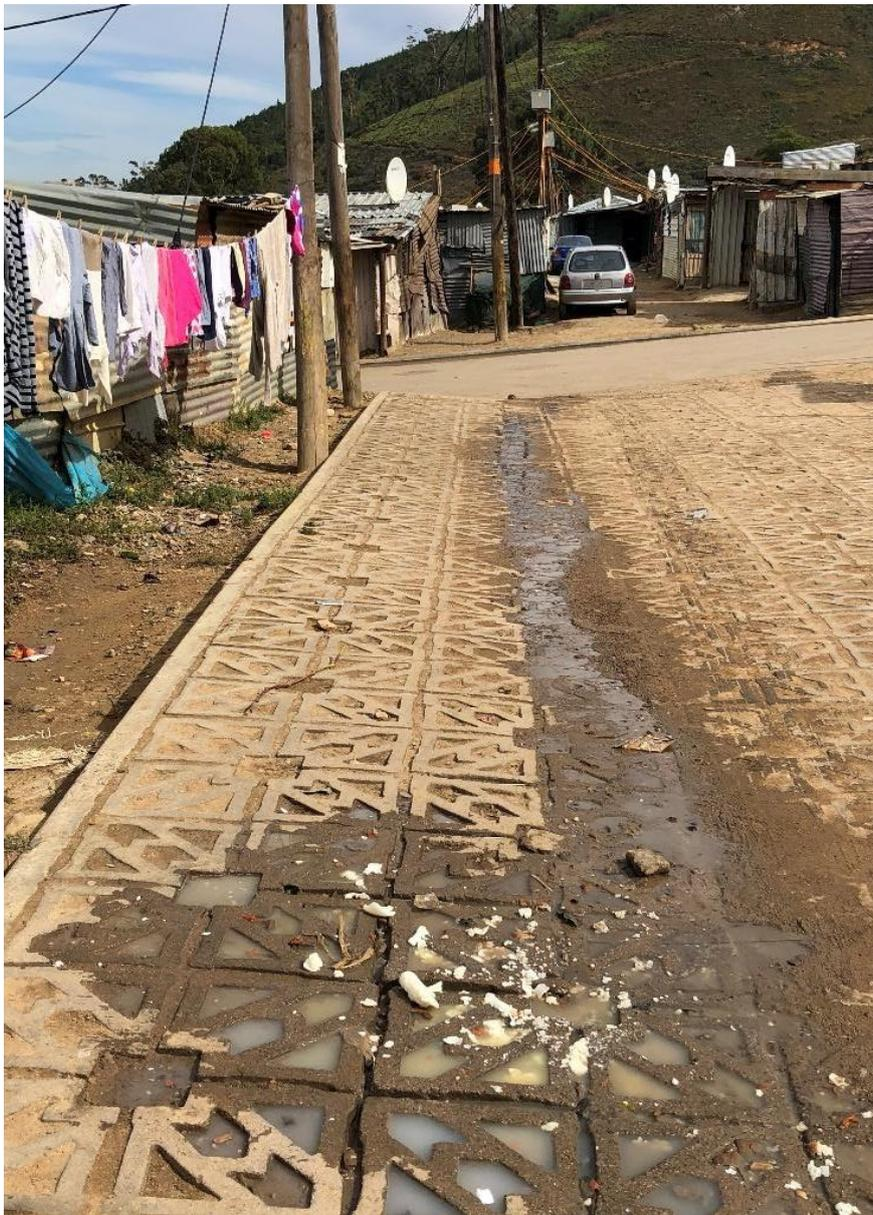
The informal community of Langrug with an improved road surface with permeable paving for stormwater management (left), and a functional greywater disposal point (blue plastic structure), Langrug (Photo credit: Alanna Rebelo).
