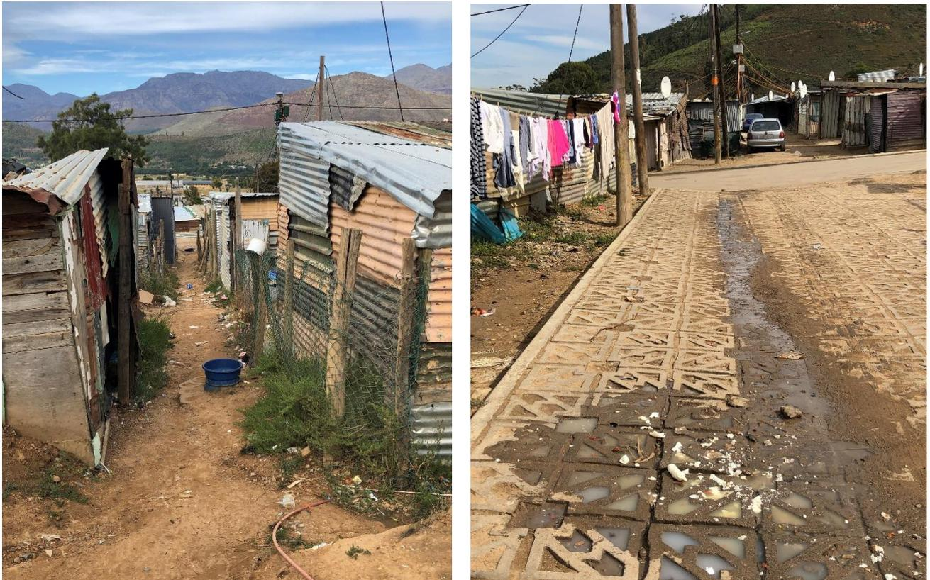
**Figure 45.** (a) An existing greywater disposal point in a walkway, also showing structures in Langrug that are typically constructed of corrugated iron sheets, and (b) An improved road surface with permeable paving for stormwater management in March 2021 (Photo credit: Karen Esler).
