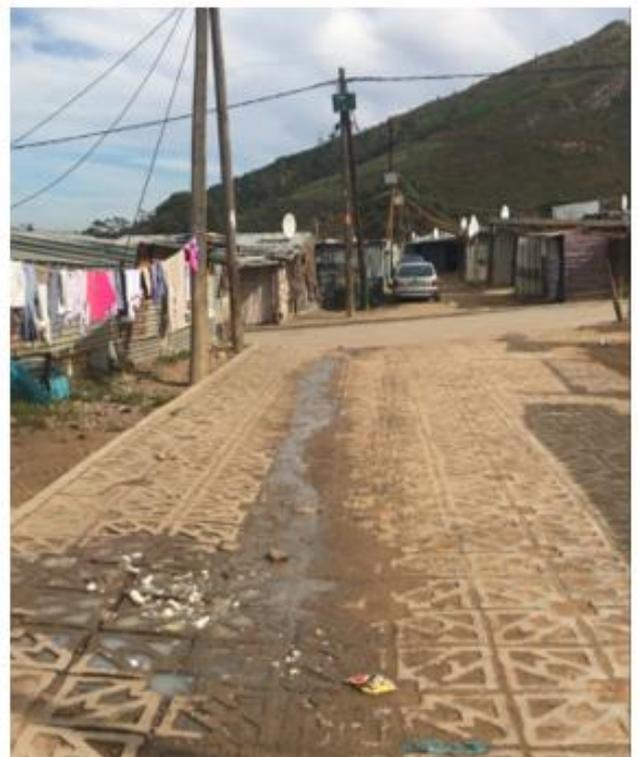
*Photo 4: Constructed permeable paving between Block S and T.*
