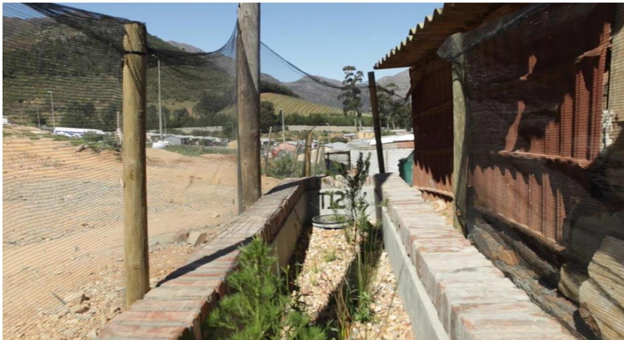
**Photo plate:** Domestic greywater treatment: Greywater flows from the disposal points through pipes to a tree garden then into “micro-wetlands” to undergo a second round of filtration and cleaning. Genius of SPACE, Langrug Community.
