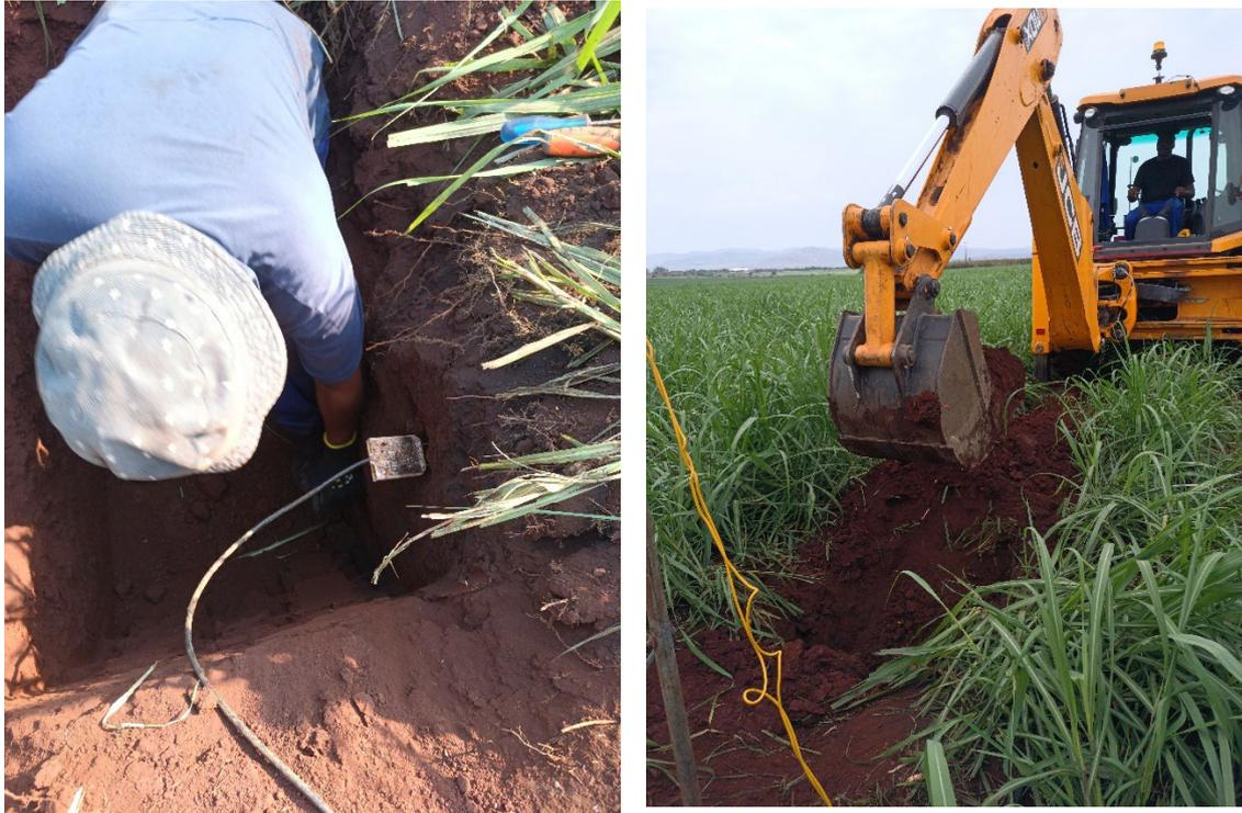
Figure 7.2: Soil Moisture probes installed at 30 and 60 cm horizontally below the ground in the profile pit.
