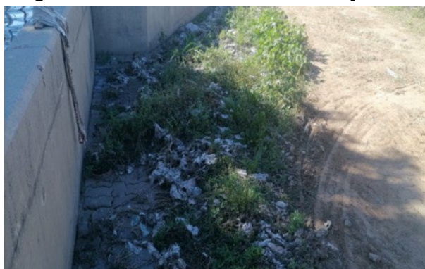
Figure 6: Screenings not safely stored
