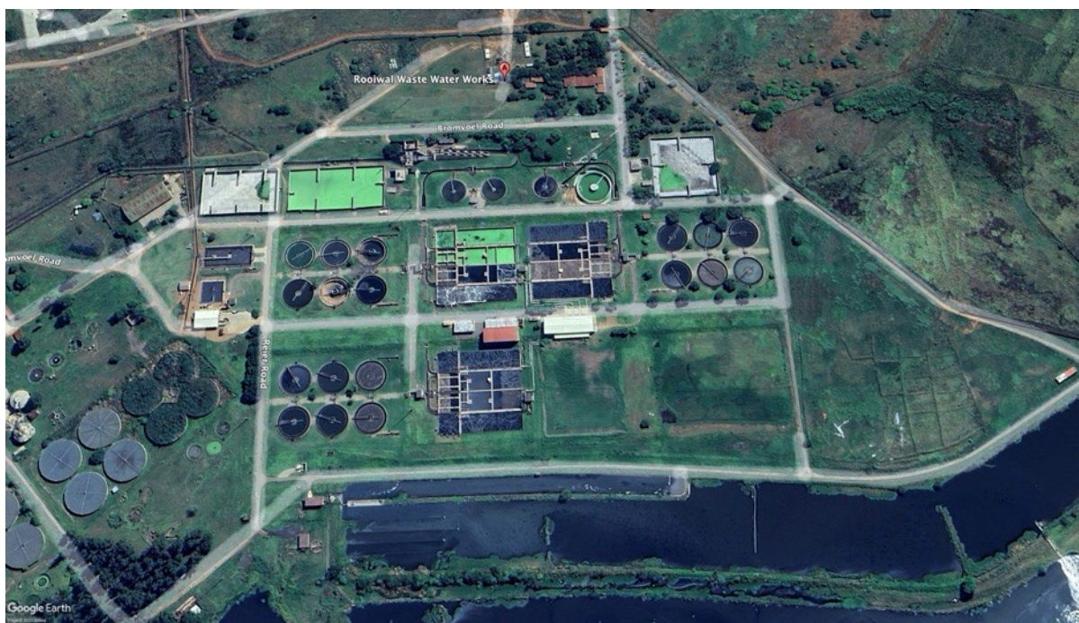
Figure 1: Aerial view of Rooiwal Northern WWTW, with clockwise from top left, Module 1, Module 2 and Module 3
