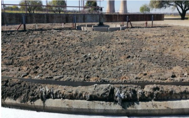
Figure 13: Typical condition of the clarifiers (module 2)
