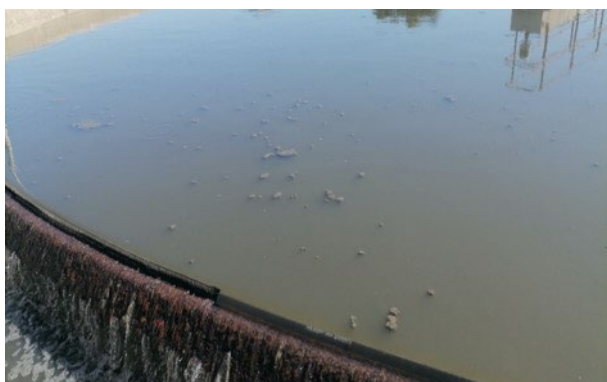
Figure 7: Sludge conditions in the PSTs
