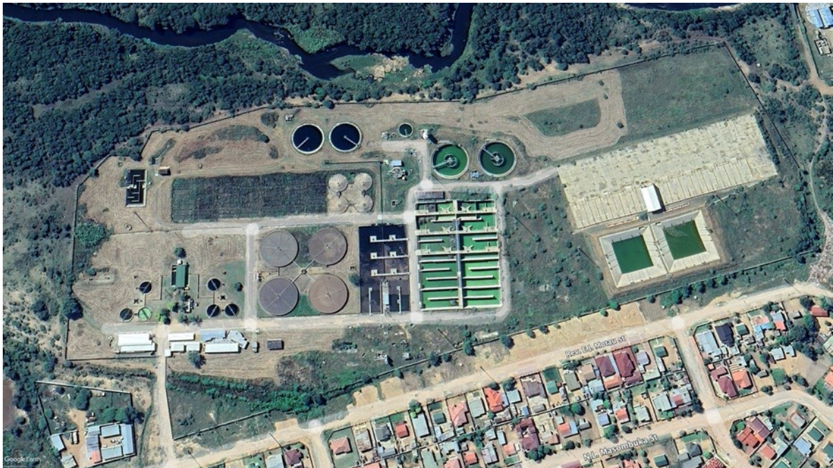
Figure 64: Aerial view of Temba WWTW (The Temba WWTW is around 25km downstream from the Rooiwal WWTW)
