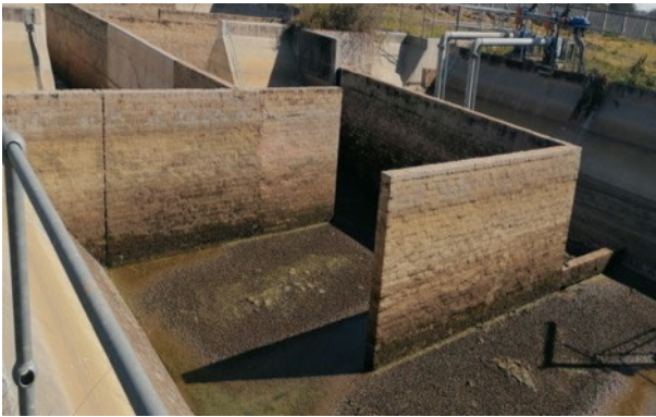
Figure 79: Contact tank isolated for cleaning
