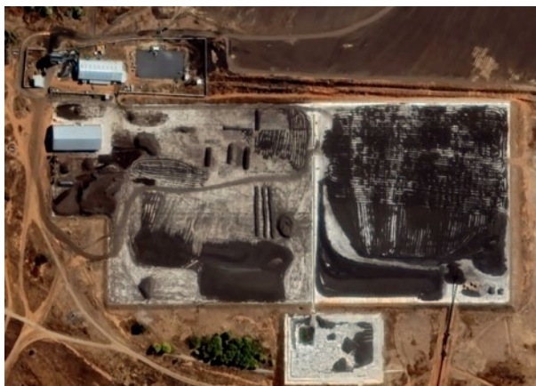
Figure 39: Dewatered sludge concrete slab c. 2015
