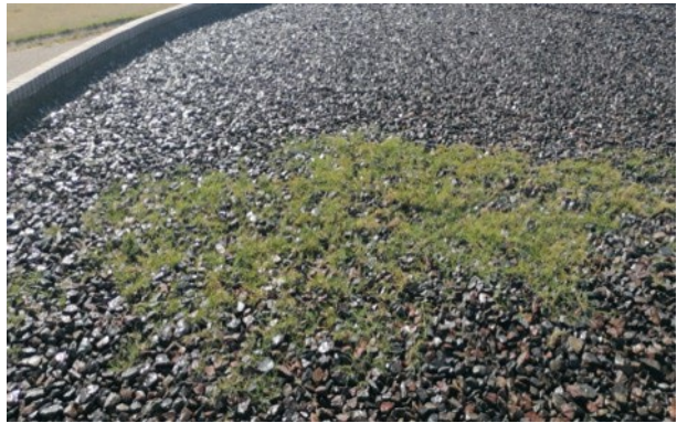
Figure 70: A patch of grass growing on the filter media
