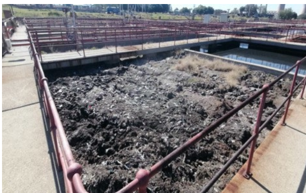
Figure 9: Typical conditions at the anaerobic zones
