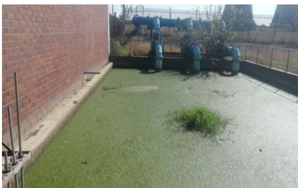
Figure 36: Duckweed observed in the final water sump
