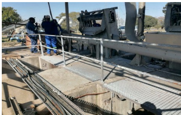
Figure 21: Maintenance team onsite to fix the screen
