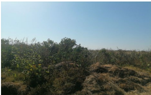
Figure 83: Excessive reeds and vegetation growth at the sludge ponds
