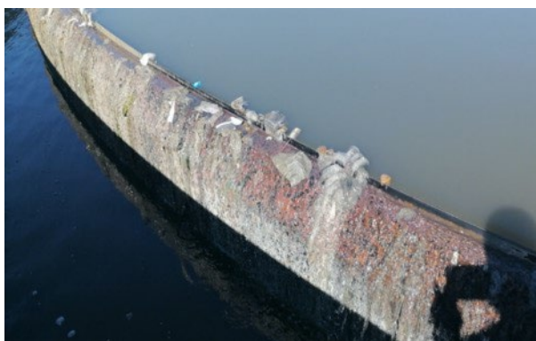
Figure 8: Debris carryover from PST
