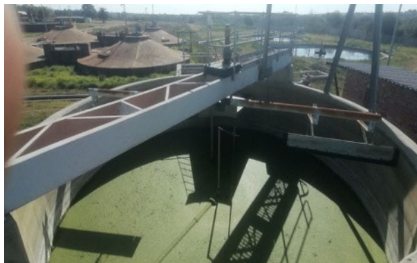
Figure 84: Presence of duckweed in the DAF unit suggests long standing time
