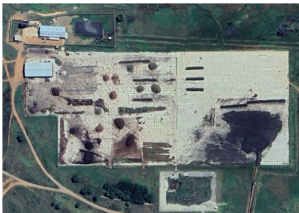
Figure 38: Dewatered Sludge concrete slab c. 2023
