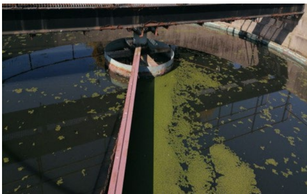
Figure 67: Traces of duckweed indicating that there was a point where the PST was out for an extended period
