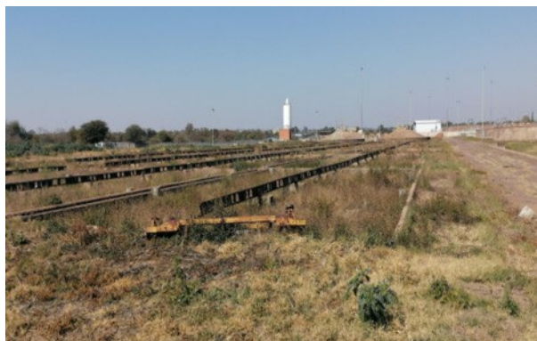
Figure 82: Poor condition of the drying beds
