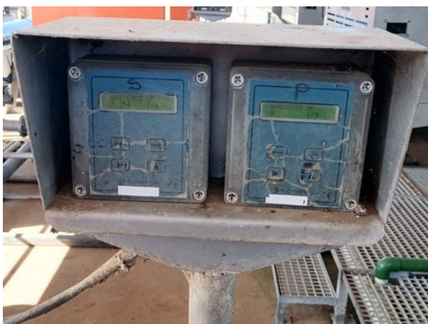
Figure 62: Sludge Flow to Dewatering Presses
