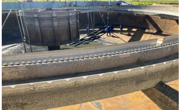
Figure 14: some clarifiers isolated for repairs (module 1)
