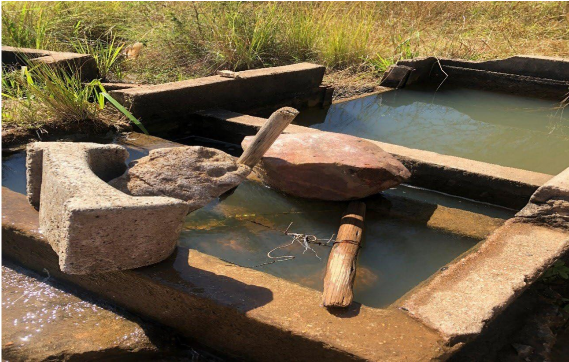
Figure 8. Major Challenges with canals at New Forest irrigation scheme
