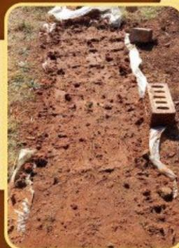
8. Plastic perforated to allow for drainage
