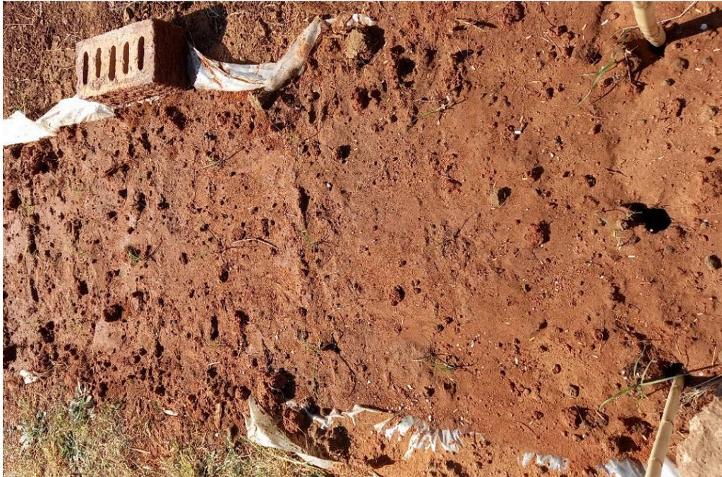
**Figure 3.2 Trap trench lined with plastic, filled with red topsoil and compost mixture.**
