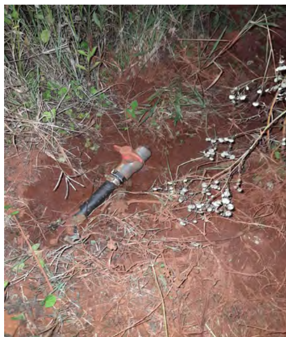
Figure 4.15: Dilapidated pipes for conveying municipal water to a farm, Thohoyandou, Thulamela Municipality
