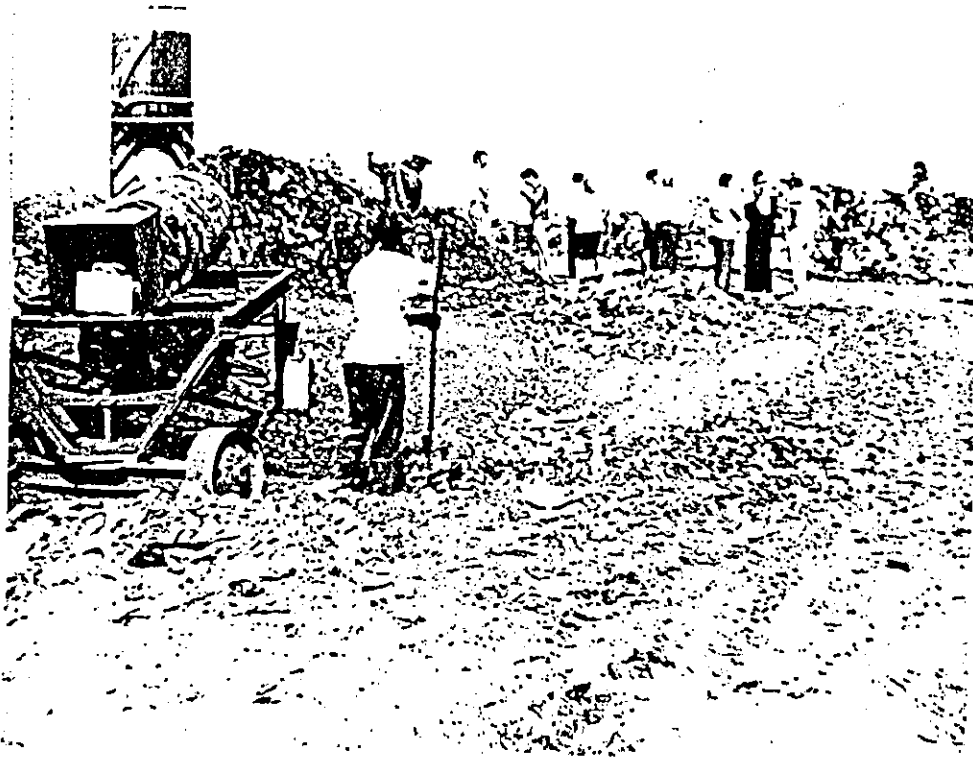
SCREENING COMPOST FROM REFUSE INERT MATERIAL.
