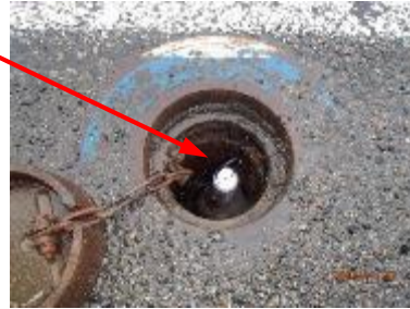
Example of the installation of a gate valve
