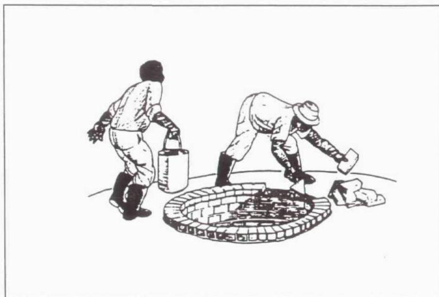
Figure 15: Finishing the pit collar
