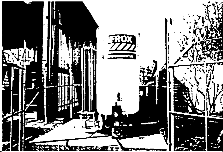
THE OXYGEN STORAGE VESSEL. CAPACITY = 1400 kg O 2 AT -186 °C. VAPORIZER UNIT IS SITUATED AT LEFT OF VESSEL
