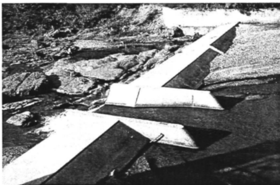
Figure 2.6: Photograph showing sluicing flume in combination with Crump weirs (Mpambanyoni River, Kwa-Zulu Natal)
