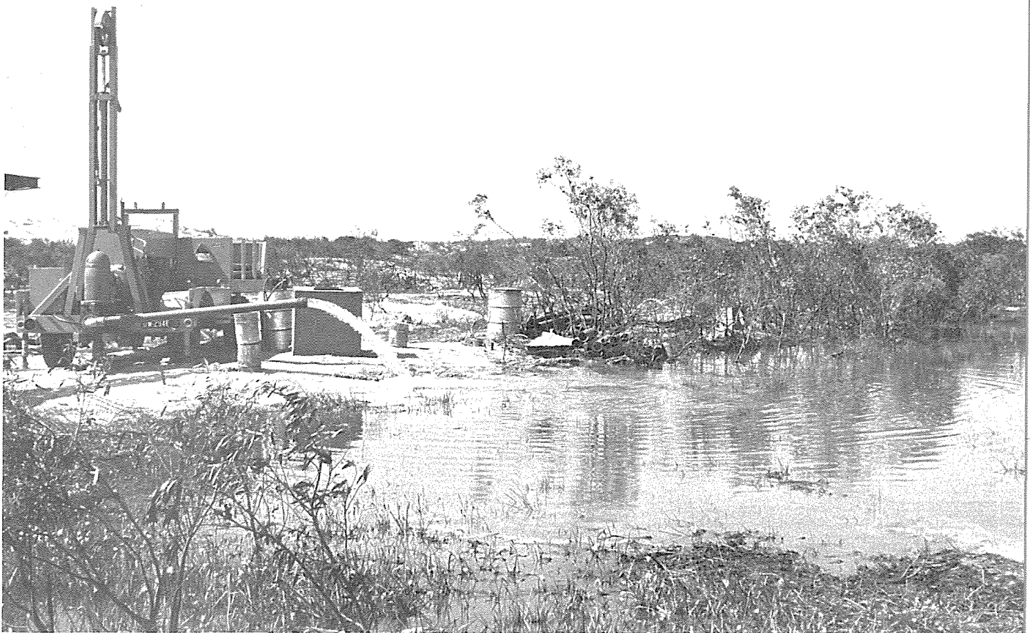
Water is pumped out of a test borehole in the sand beds of the Cape Flats at a rate of 4,5 Ml a day, evidence that it is possible to store a considerable volume of water in the sand and extract it as required.
