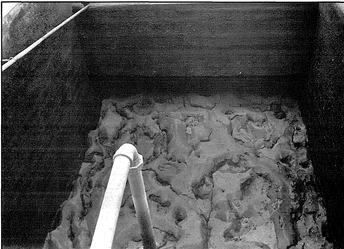
Sludge originating from the water purification process. Disposal of the sludge creates problems and is now being investigated.
