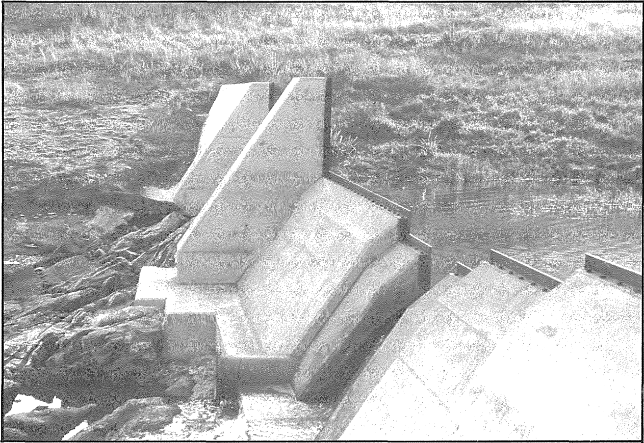
A weir in the Mtunzini catchment being used for studying runoff in small catchments.
