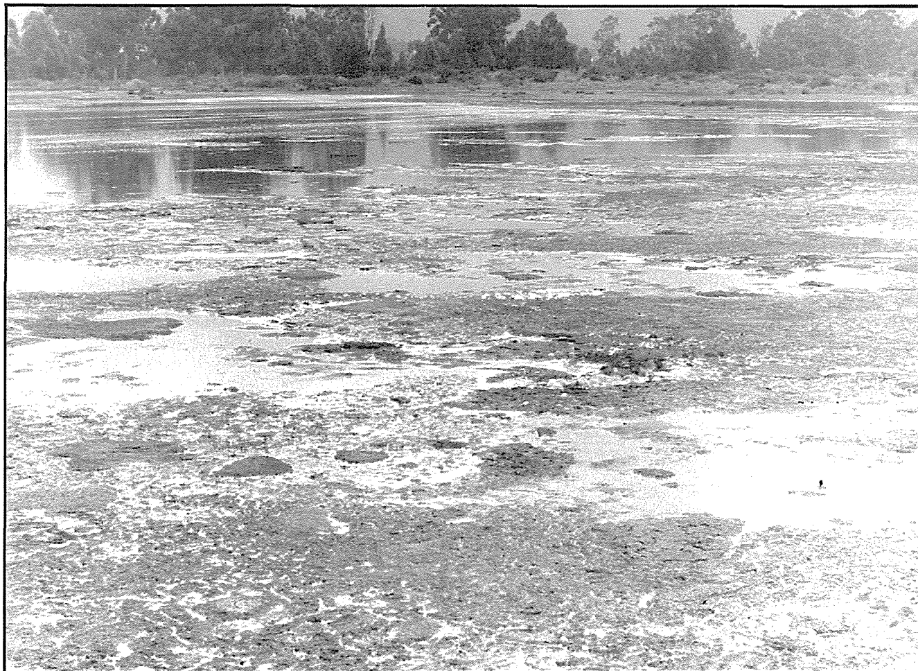
A typical storage dam for scouring effluent at a commercial wool scouring concern. The layer of grease covering the water surface is clearly visible. The Chemical Engineering Department of the University of Natal is investigating methods for treating this highly polluting effluent.
