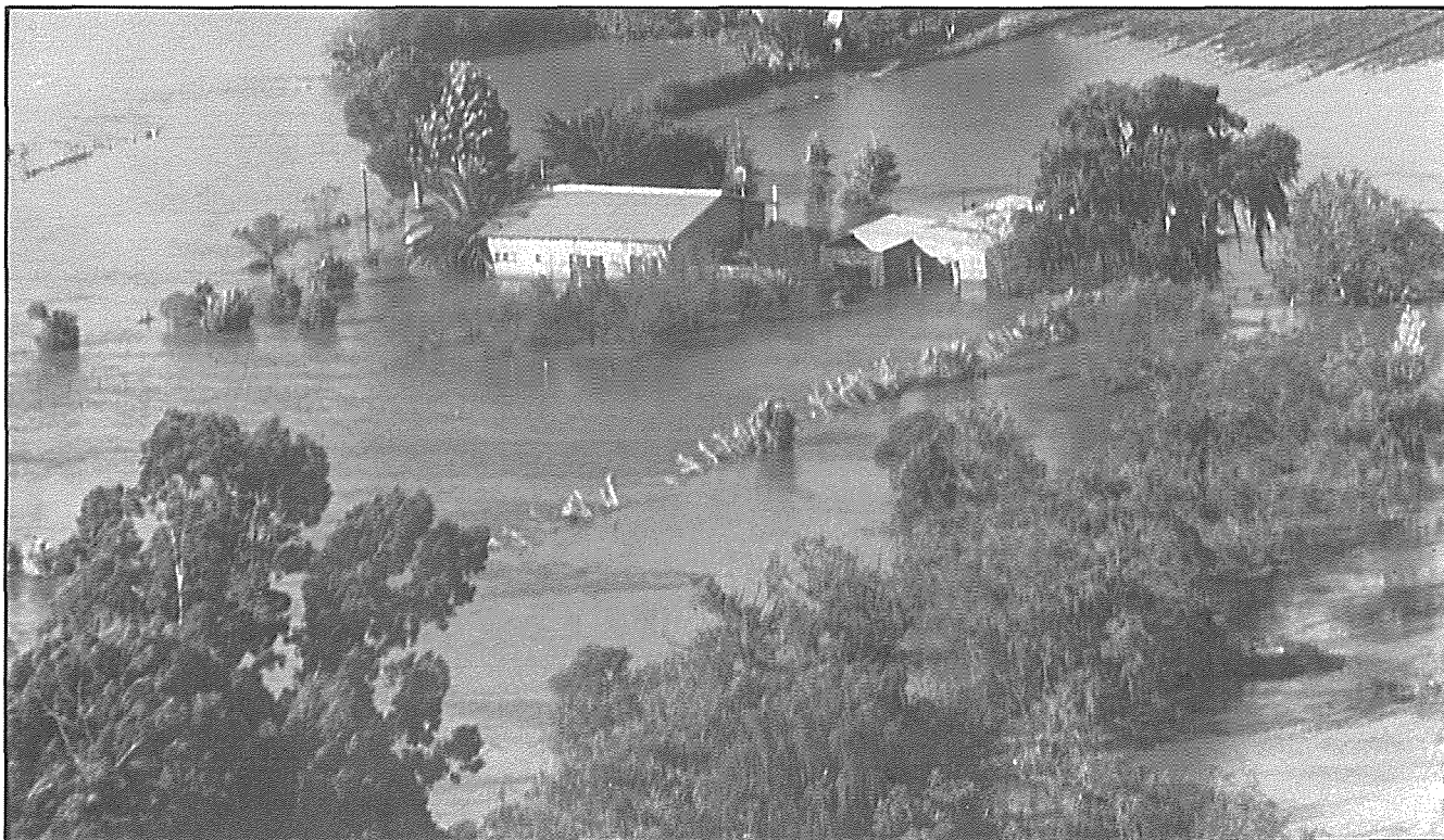
A characteristic flood scene after a severe storm. The Water Research Commission supports projects on flood damage and occurrences
