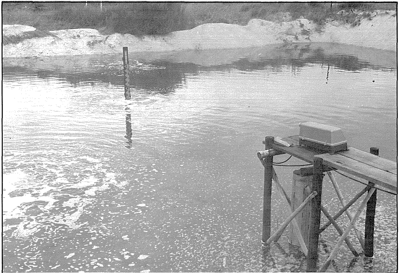
An infiltration pond in the sand deposits of the Cape Flats
