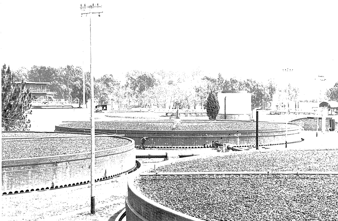
Biological filters at the Daspoort sewage works where research was conducted on chemical phosphate removal from effluents.
