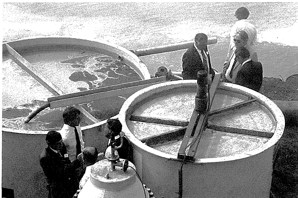
A dissolved air flotation unit used for the treatment of fish processing effluent in St Helena Bay.
