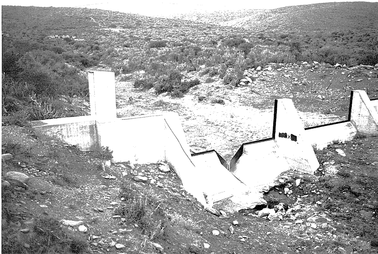
A weir which was used for hydrological research in the Eccca catchment.
